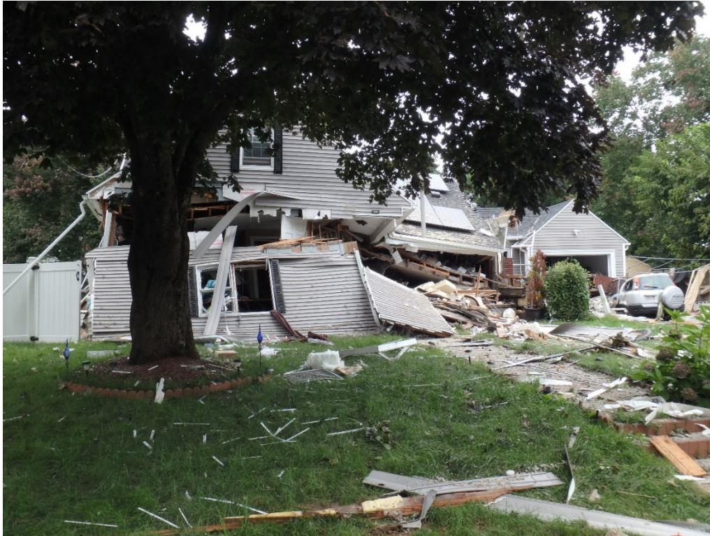
Figure 2. Remnants of house where the fatality and two severe injuries occurred.
