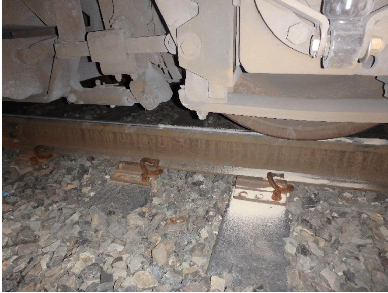
Figure 2-Sand on rail and under the front left wheel from locomotive 4214
