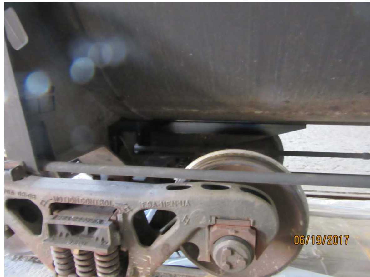
Figure 4228: TILX 199545, tank support structure and truck mount
