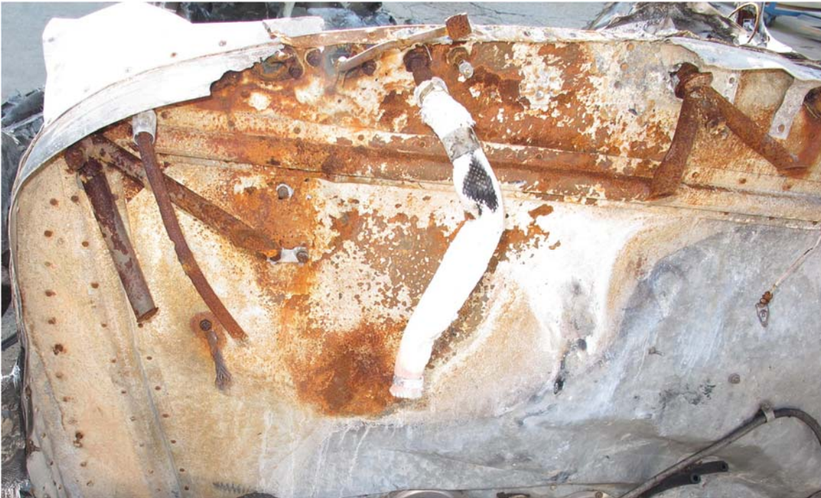
Figure 10. Closeup photograph of clean burn area.
