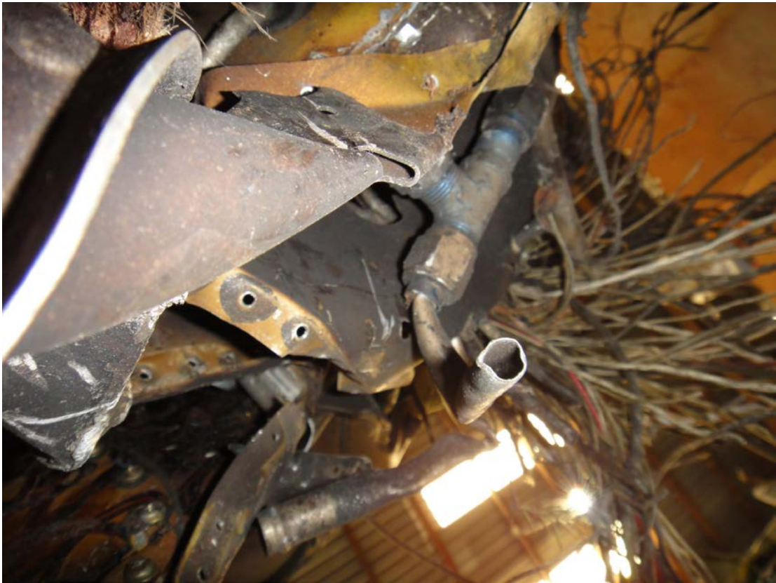
Figure 17. Closeup photograph of fuel crosstie lines at wing spar.
