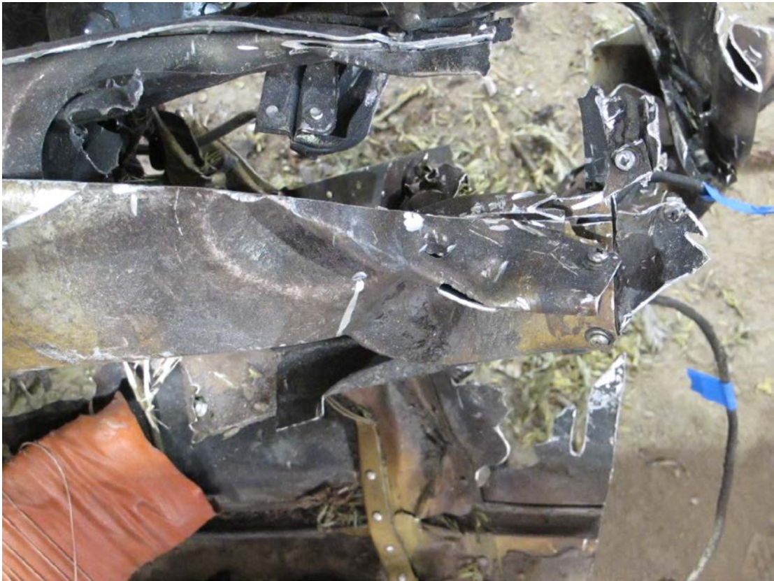
Figure 10. Photograph of thermal damage to aircraft structure near main bus tie circuit breaker panel.
