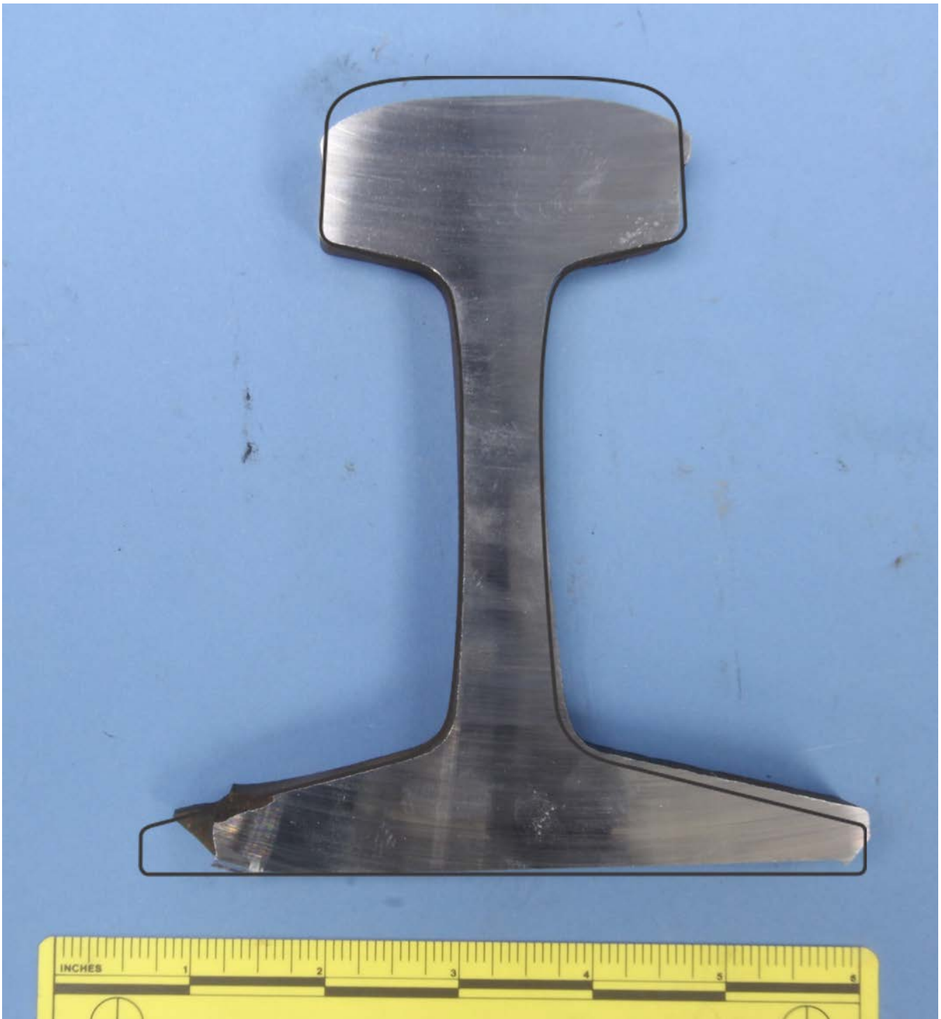
Figure 39 – Cross section through piece 10N with an outline profile of a new 90-pound rail for reference.
