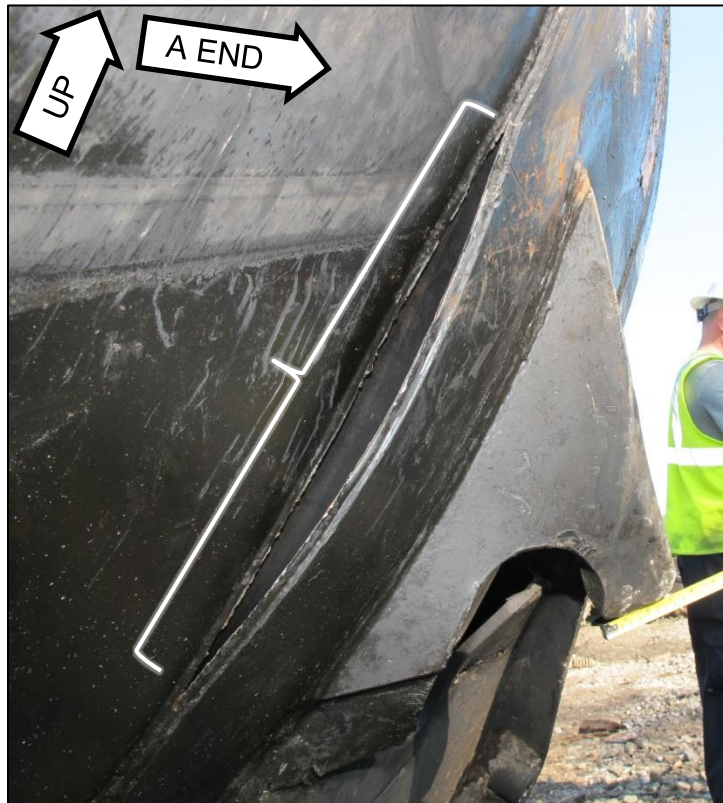
Figure 10. The weld at the B side of the body bolster pad was fractured in the area indicated with an unlabeled bracket.
