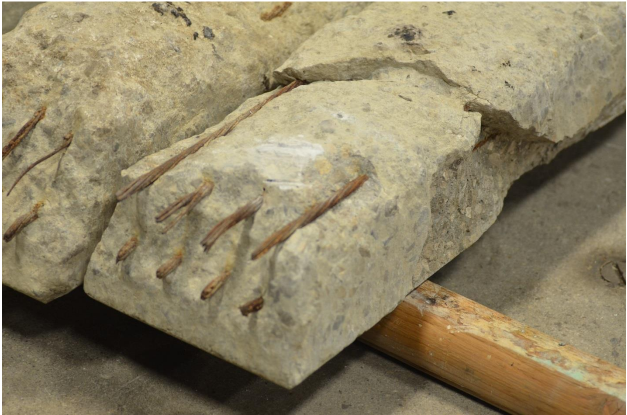
Figure 6. View of freshly broken off concrete area on Specimen S4.
