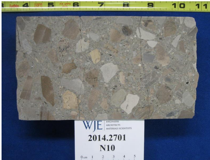
Figure 5. Core N10. Lapped cross section illustrating the appearance of the concrete. In-service top end is on left.
