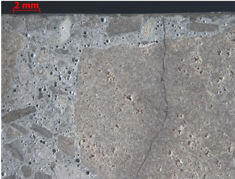
Figure 9. Core NEW. Close-up view showing vertical crack passing through a coarse aggregate particle, and example of air-void system in the near-top region. Epoxy was applied to the crack surfaces to reassemble the core.
