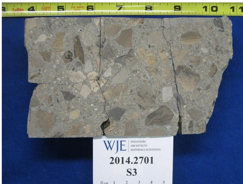
Figure 2. Core S3. Lapped cross section illustrating the appearance of the concrete. In-service top end is on left.
