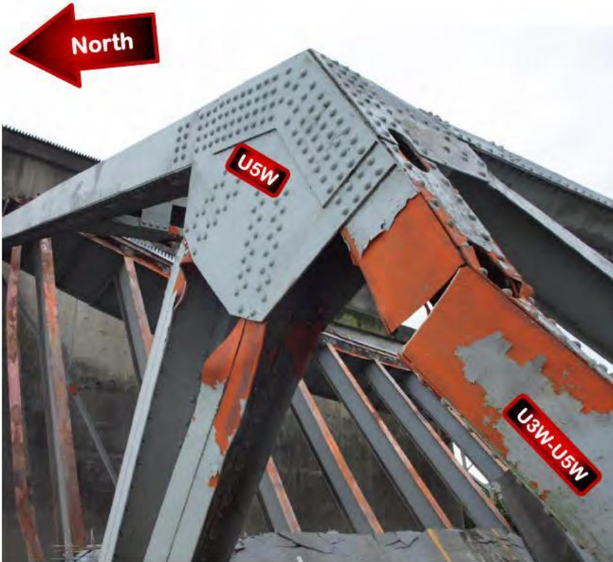
Figure 10. Top, an overall view of node U5W with a view of overstress fractured member U3W-U5W below.
