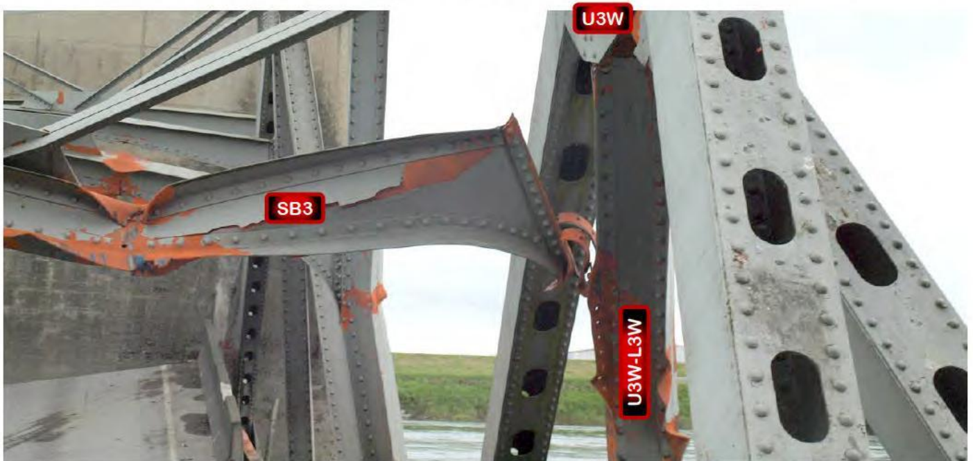
Figure 17. Upper view shows impact damage to sway brace 3 in the foreground along with impacts on SB2, 1 and 0 in the background. Separation of SB3 from vertical U3W-L3W is depicted below. Both views looking south.
