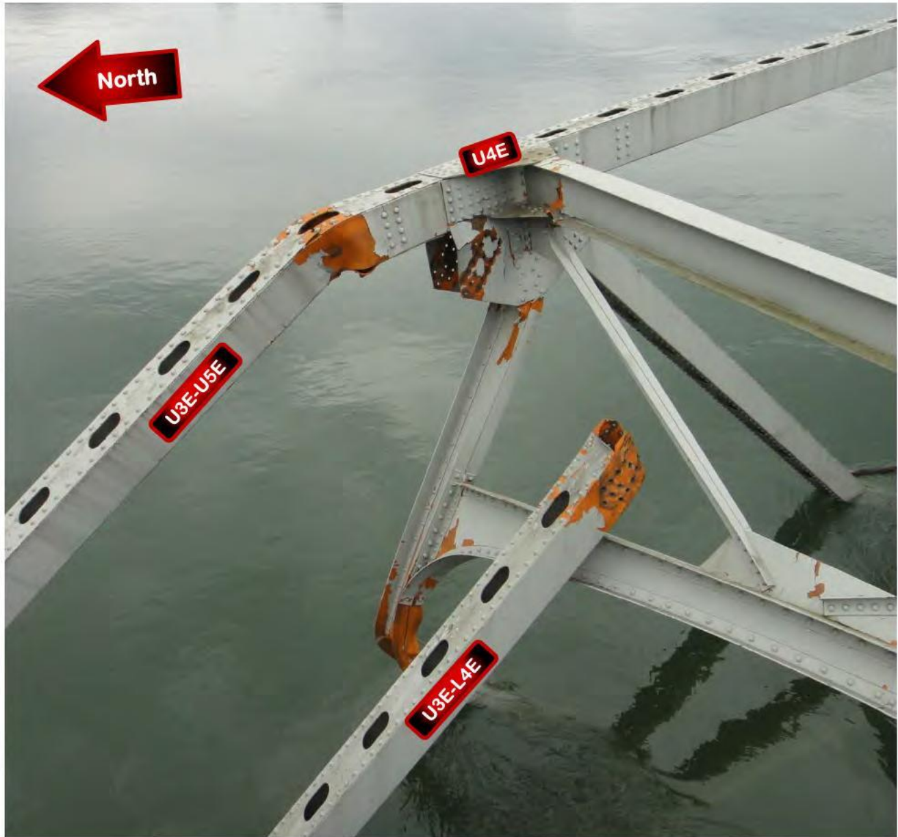
Figure 11. Node U4E with separated member U3E-L4E.
