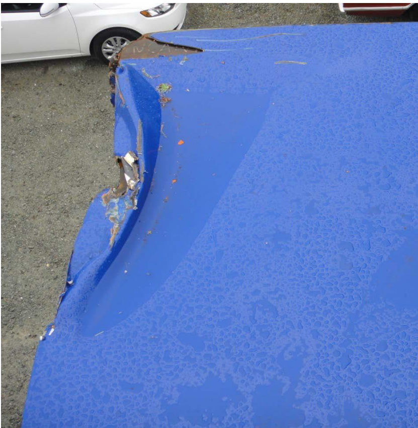
Figure 30. Closer view of the damaged area (boxed area from figure 29) from the front (top view) and top (left view).
