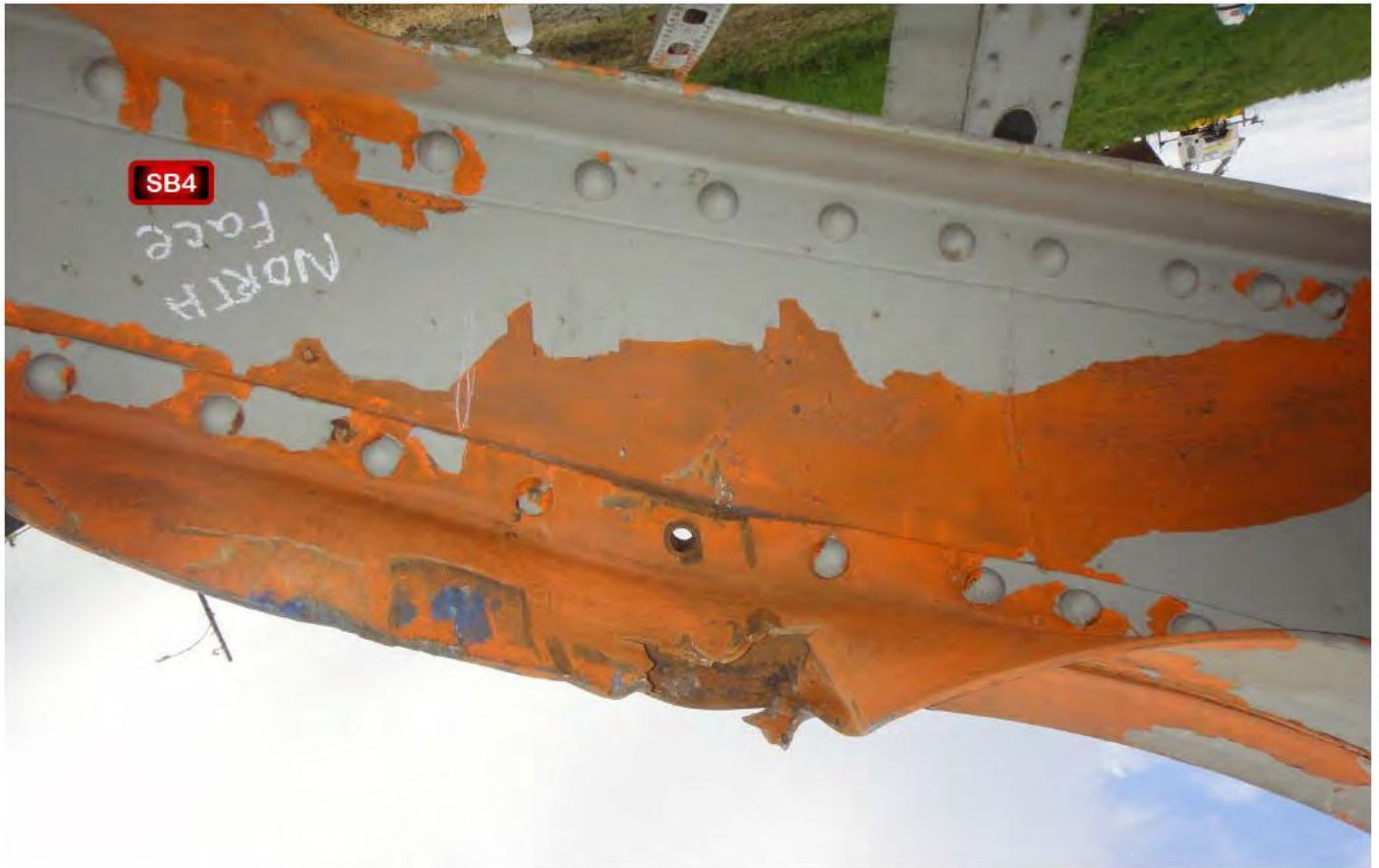
Figure 16. Impact damage to sway brace 4 above with extent of bowing depicted below.
