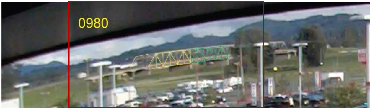
Figure 2. The cropped image from figure 1 with the visible members of span 8 trusses denoted in yellow. The red line indicates the north portal. Identified members of span 7 are highlighted in green. Red box indicates the additional cropping used for display in this report (see below).
