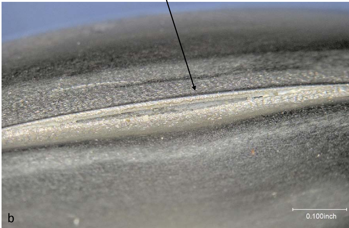
Figure 6 View (a) showing a dent on the surface of the float and a fracture in the solder joint. View (b) is a closer image of the solder joint fracture.
