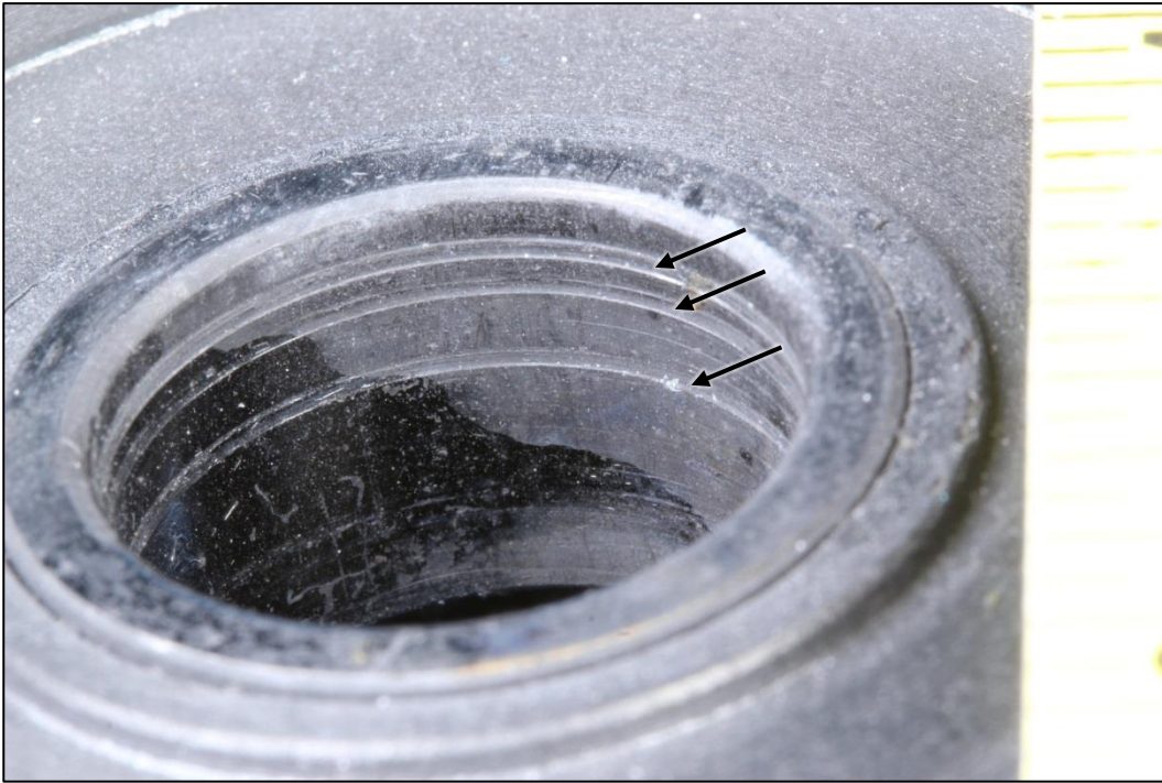
Figure 6. Circumferential score marks in the drive shaft bearing.. Unlabeled arrows point to the score marks.
