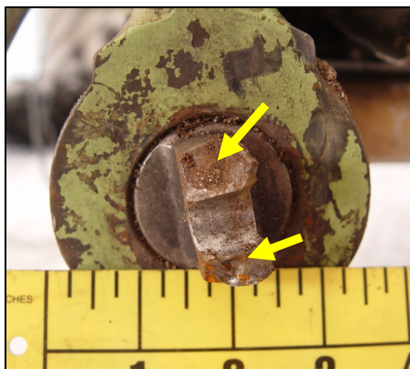
Figure 29. The inboard forward engine attachment indicated by the purple arrow in Figure 27 and in Figure 5.
