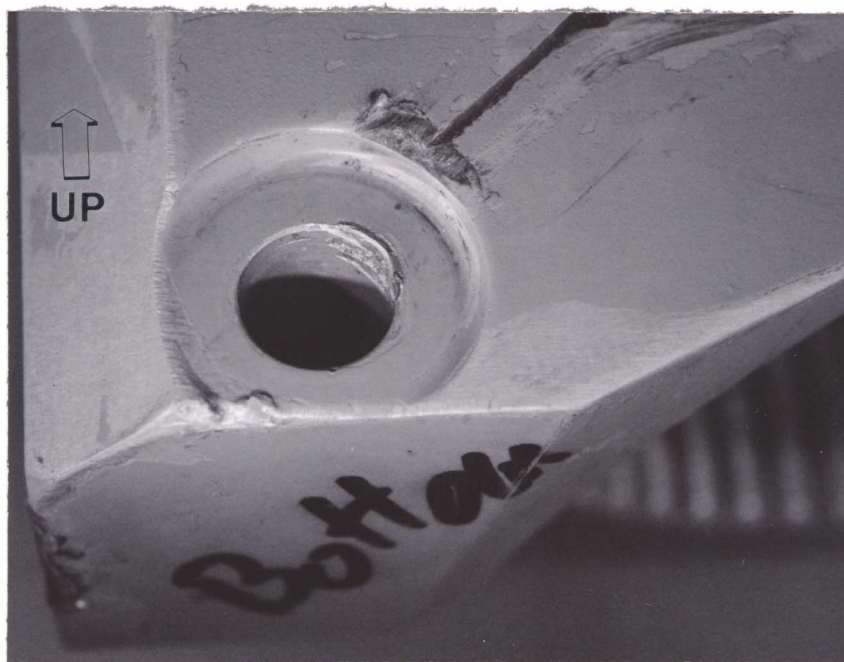
Figure 21. A higher magnification view of the nut end of the stop bolt hole "n" shown in figure 20. Thread impressions are shown in the hole for the stop bolt. (3.3x)
