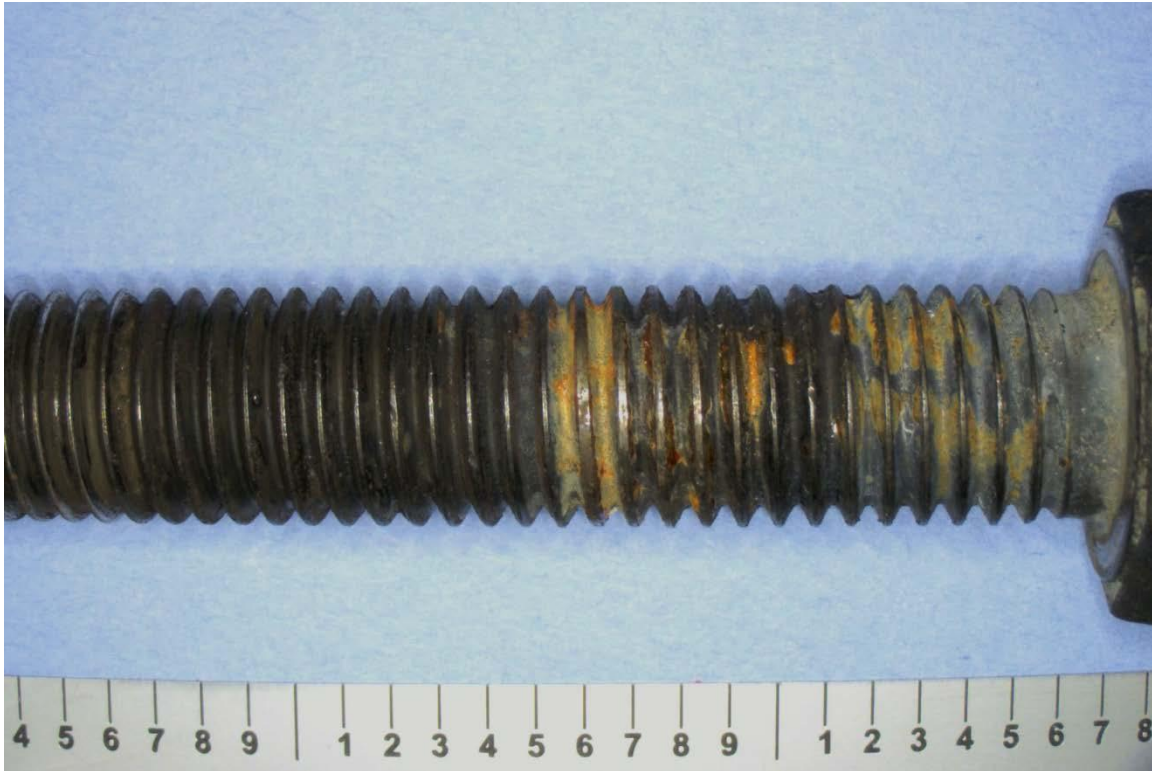
Figure 1. Fuel pump housing bolt found attached to housing.
