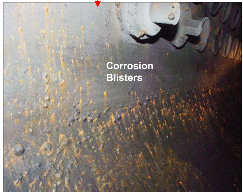
Figure 8: Views of selected areas of the interior of headers 21 and 24.
