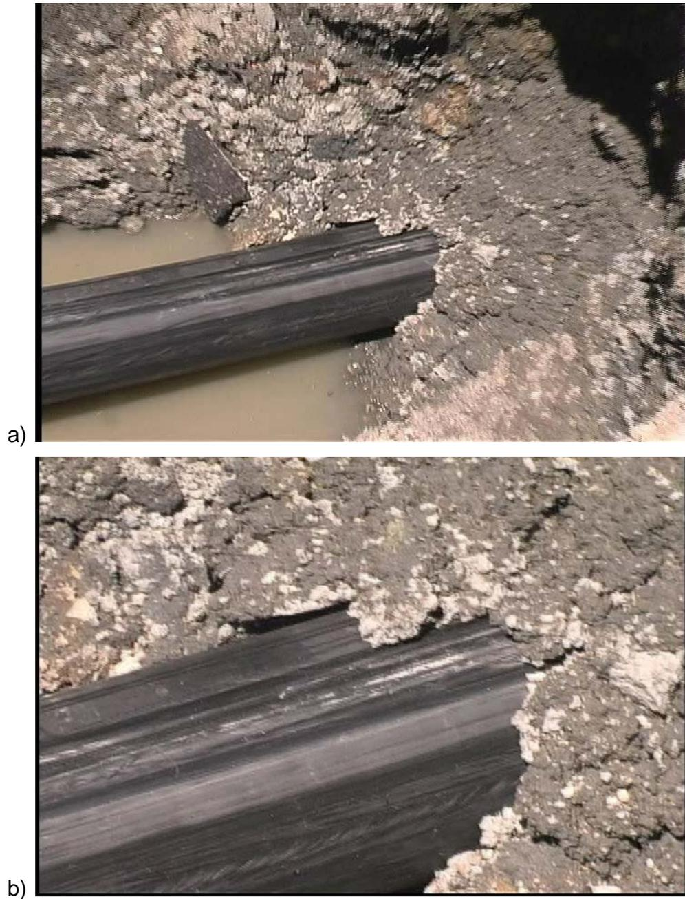
Figure 5: Video frames of the sewer pipe as it entered the ground at the insertion pit. The frames were separated by 4.80 s. The images were calibrated using the diameter of the sewer pipe (10 inch).
