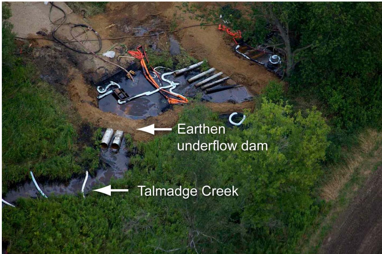
Figure 10. Underflow dam on Talmadge Creek on July 30, 2010.
