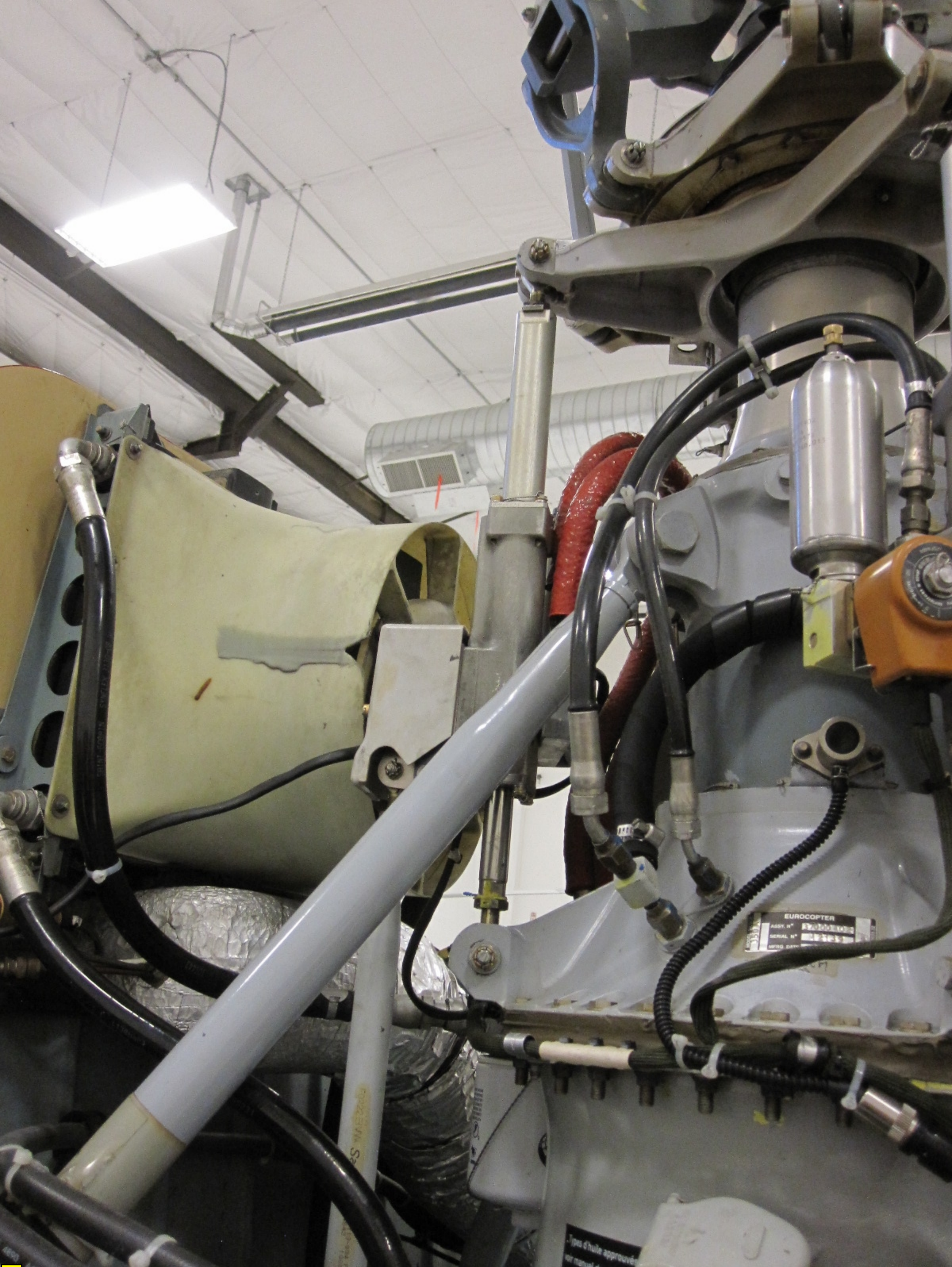
Maintenance 11 - Photo 1. Input Rod Installed
