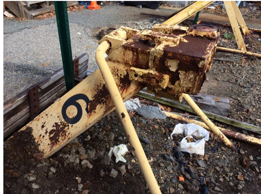
Western Railroad Supply Port Washington TK 6
