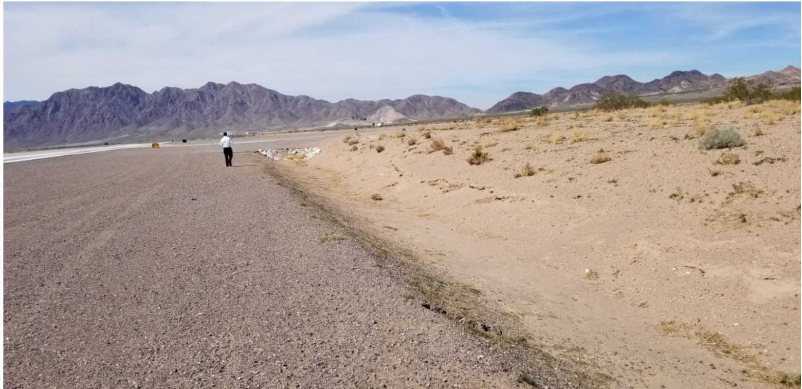
Figure 2 - Tire Track Marks and Ditch
