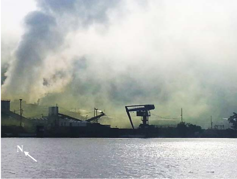
Figure 13: Water vapor from a cooling tower rises nearly vertical with a slight tilt to the south. The green to yellowish lower cloud is the visible indication of the chlorine release. August 27, 2016 (courtesy West Virginia Division of Homeland Security and Emergency Management)
