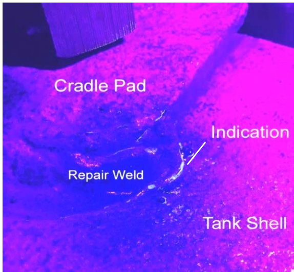
Figure 18: Wet magnetic particle examination at termination of right B end cradle pad (A6) fillet weld, with indication at toe of the weld, November 9, 2016.
