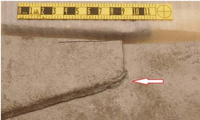
Figure 19: AXLX1702 B-end stub sill weld termination ultrasonic testing scan area, November 9, 2016.
