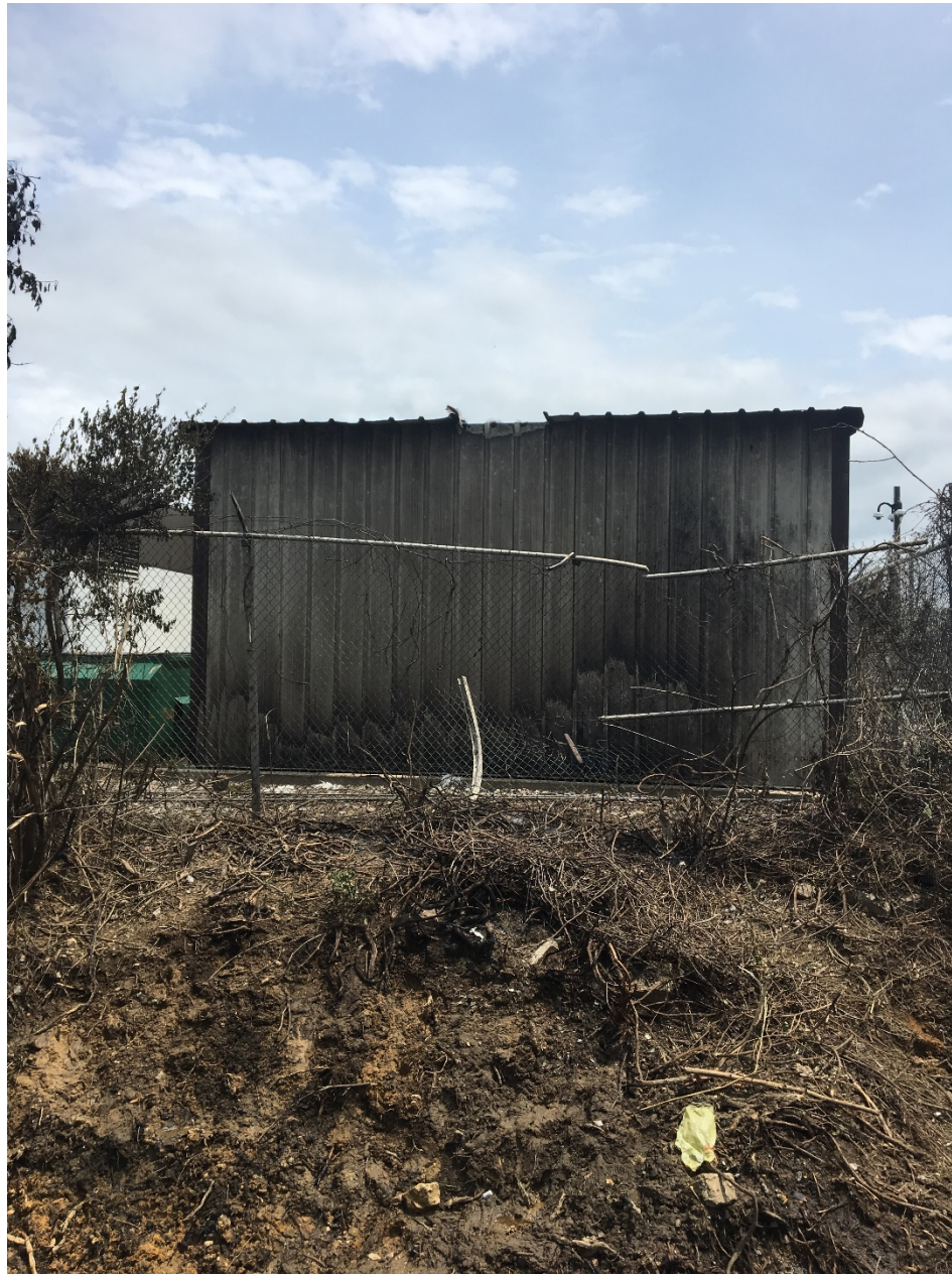
Photo 3 – Fence with cut
