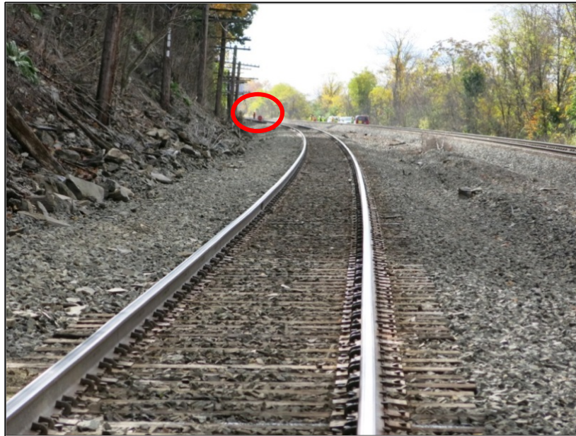
Figure 1. A ground level view looking south at main track 1 at the curve north of accident site. The red circle indicates location of employees at 100.9 2 .
