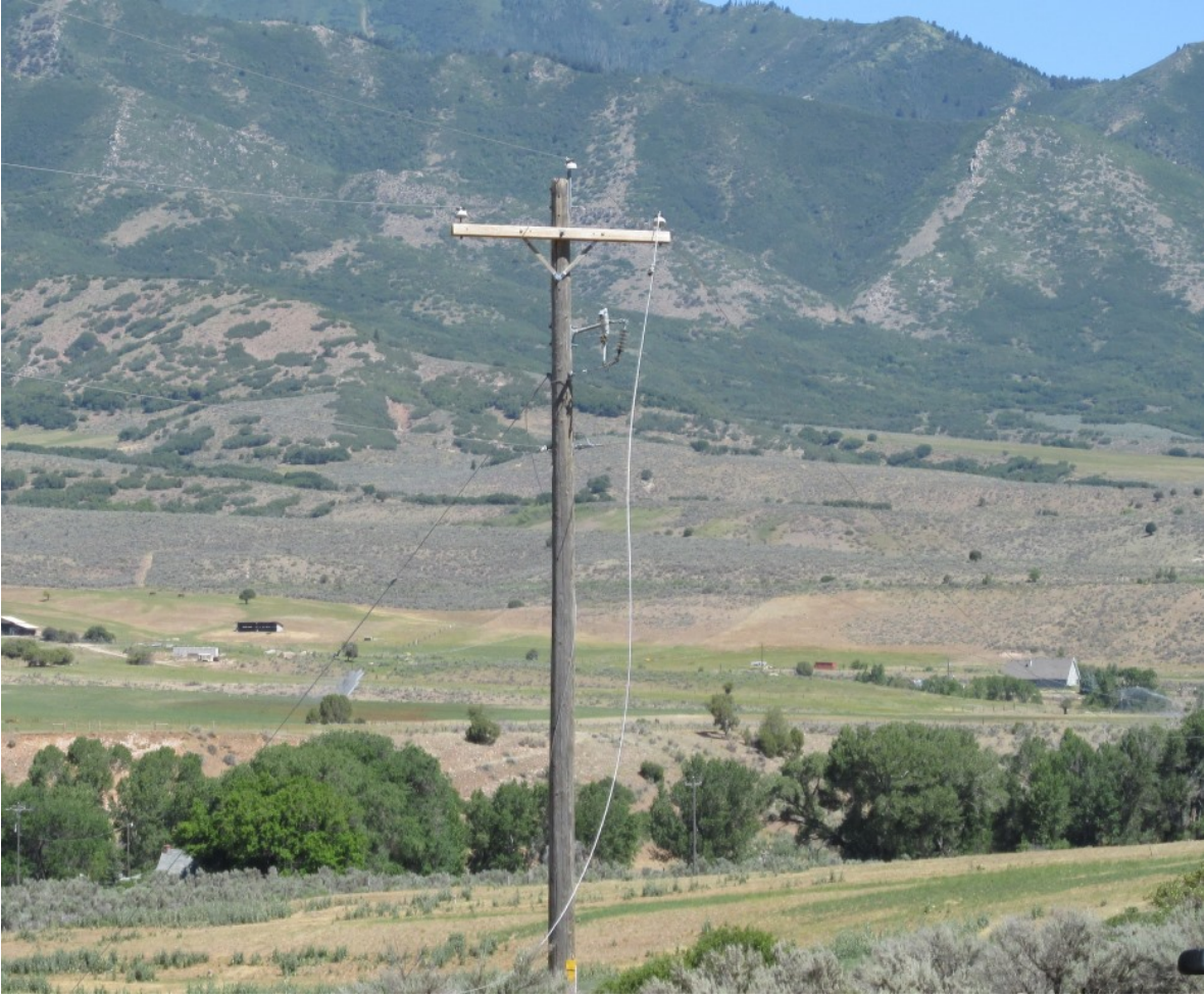
Figure 10 – Pole Supporting Parallel and Transverse Powerlines
