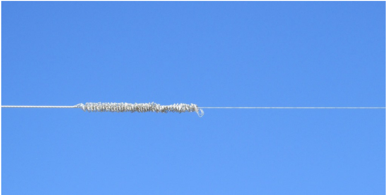
Figure 9 - Bunched Wires on Parallel Powerline
