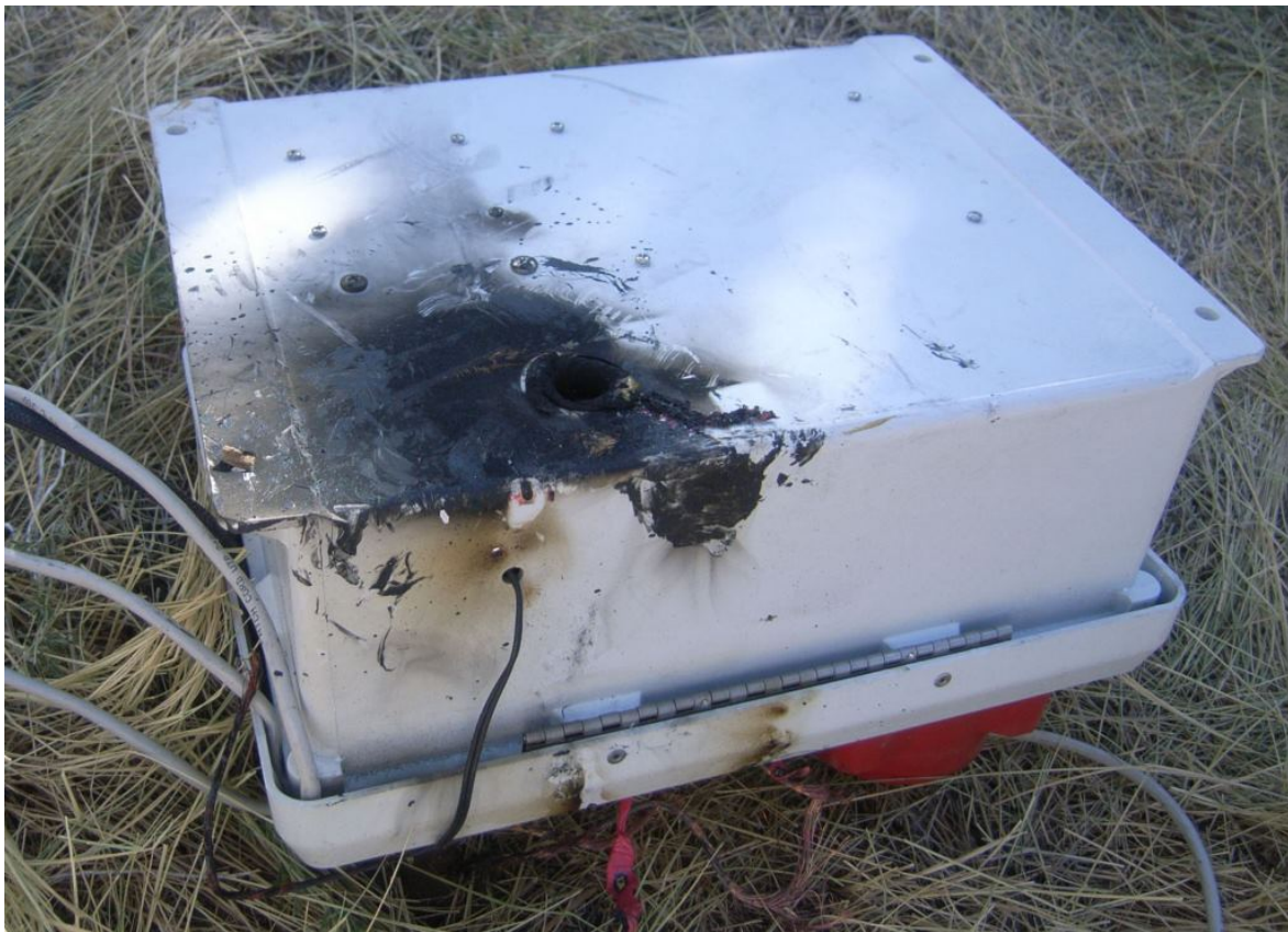
Figure 40 - Underside of Distribution Box
