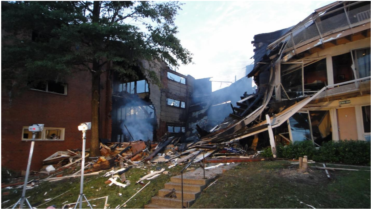
Figure 1: Buildings 8701 (right center) and 8703 (left), Arliss Street, Silver Spring, Maryland, after the explosion and fire. (Photo provided by Public Service Commission of Maryland)
