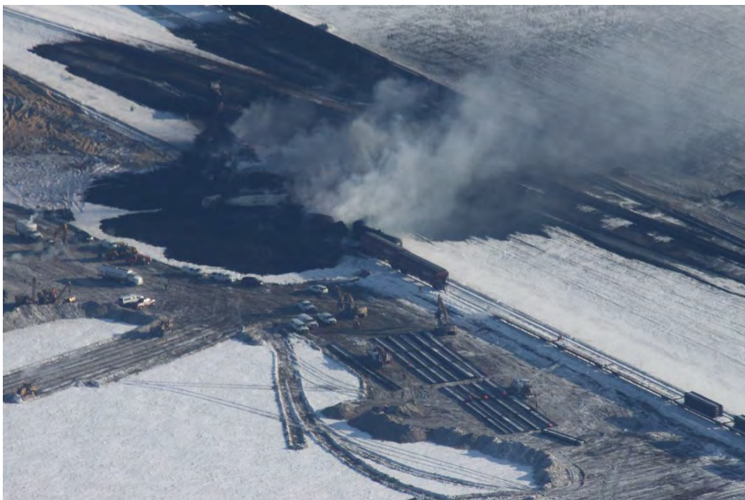
1 2 Figure 57. This is an aerial image of derailment taken from the northwest. 21
