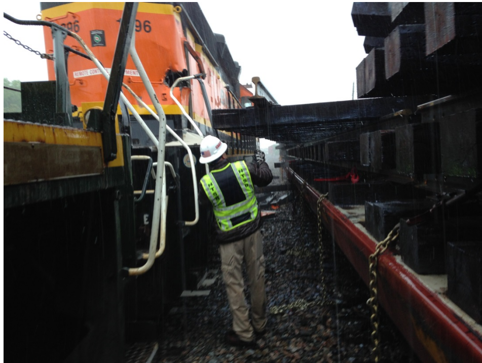
Figure 6. This is a view of dislodged track panel and damage to front end of trailing locomotive BNSF 1896.
