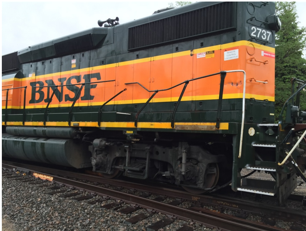
Figure 4. View of the south side of locomotive BNSF 2737 showing damaged hand rails.
