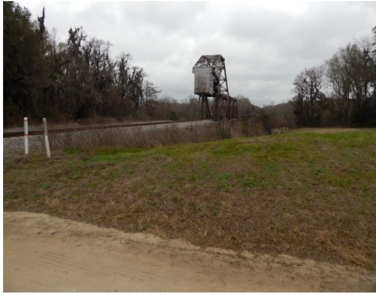
Figure 1. Railroad bridge over the Altamaha River. (Photo by CSX)
