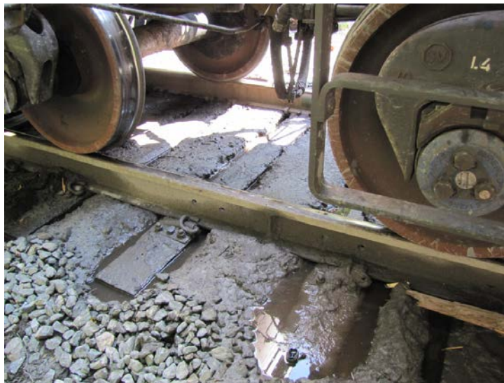
14 15 16 Figure No. 7. View of water and mud condition under derailed car.
