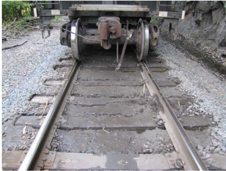
Figure No. 8. View of a fouled ballast condition
