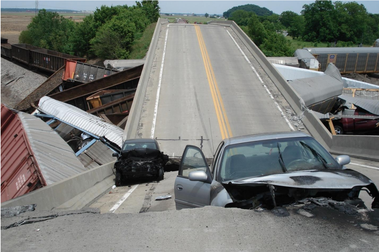
3 4 Figure 5: Collapsed bridge deck
