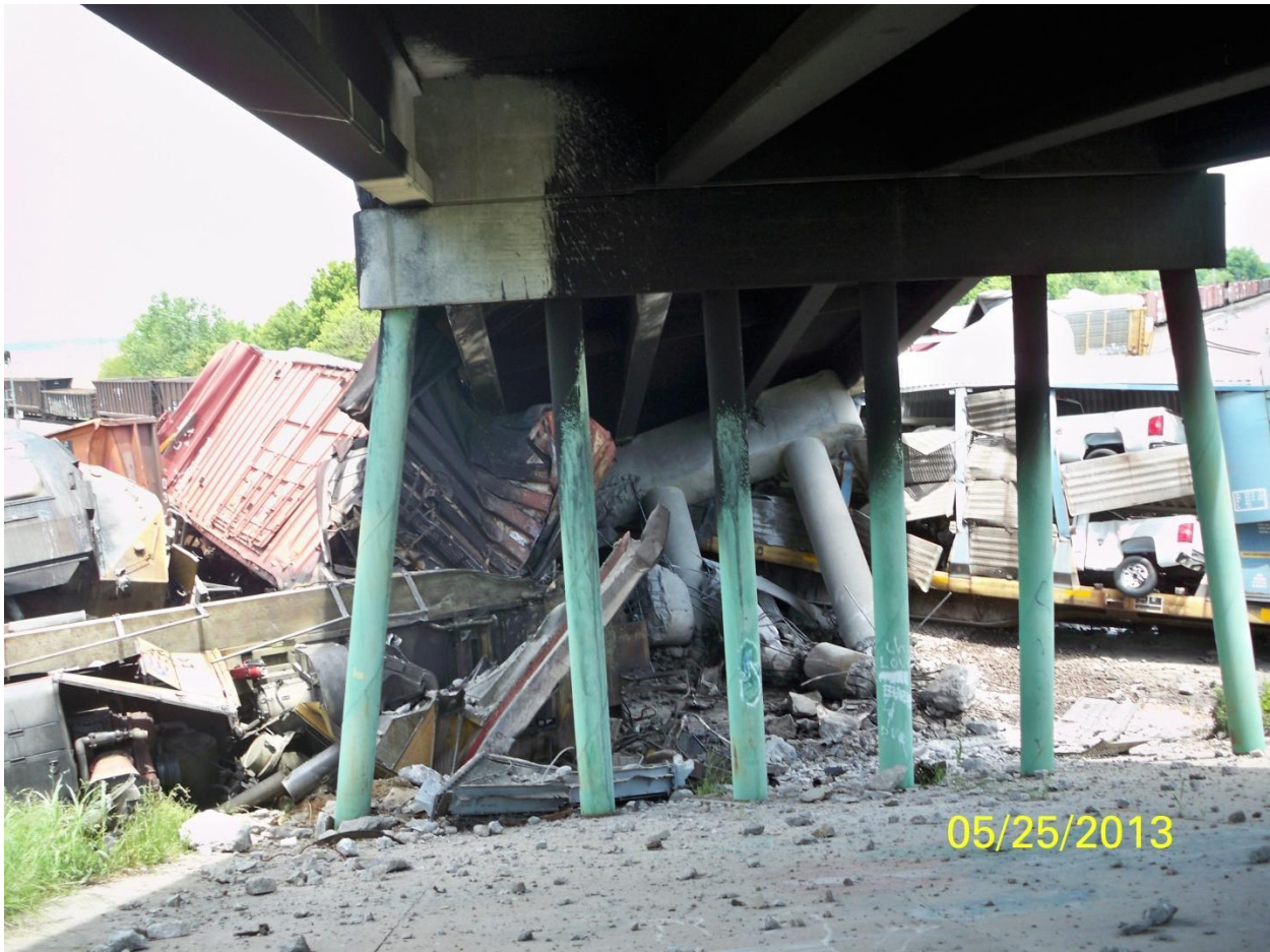
2 Figure 4: Derailed cars and damaged bridge supports
