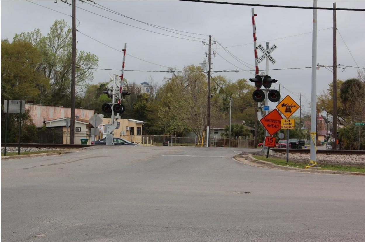
Figure 2. View of Crossing from Motorcoach Approach Direction
