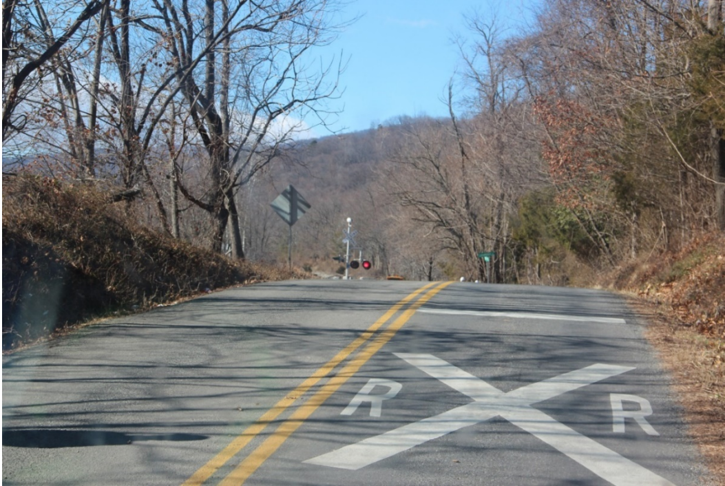
Figure 1. Illuminated Crossing Light Visible from Exemplar Truck
