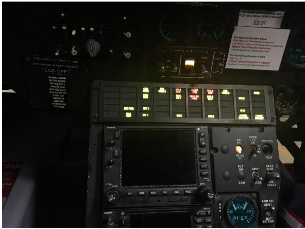
Photo 2. Caution/warning panel; instrument lights set to “OFF”; transfer pumps “OFF”; taken in hangar with hangar lights on.
