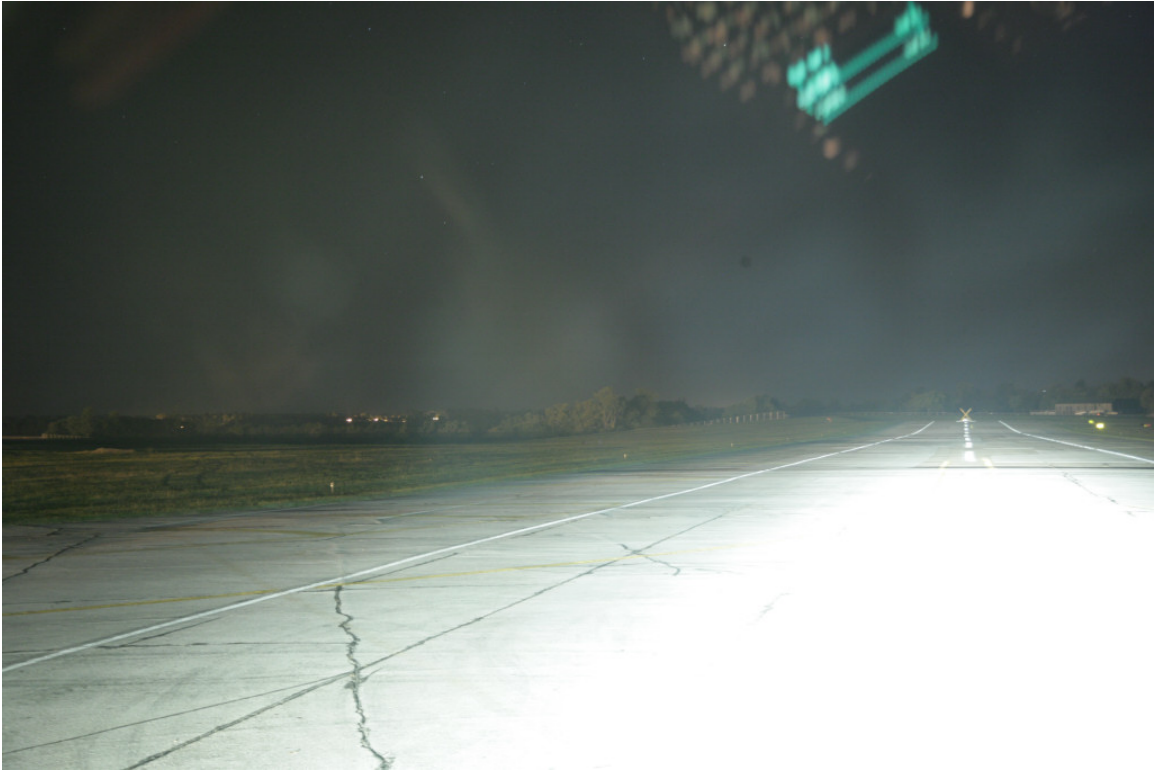
Figure 9. Position 11 – Forward left view down RW26. (Image is overexposed. Horizon, end of RW, RW closed "X", other structures were not visible.)
