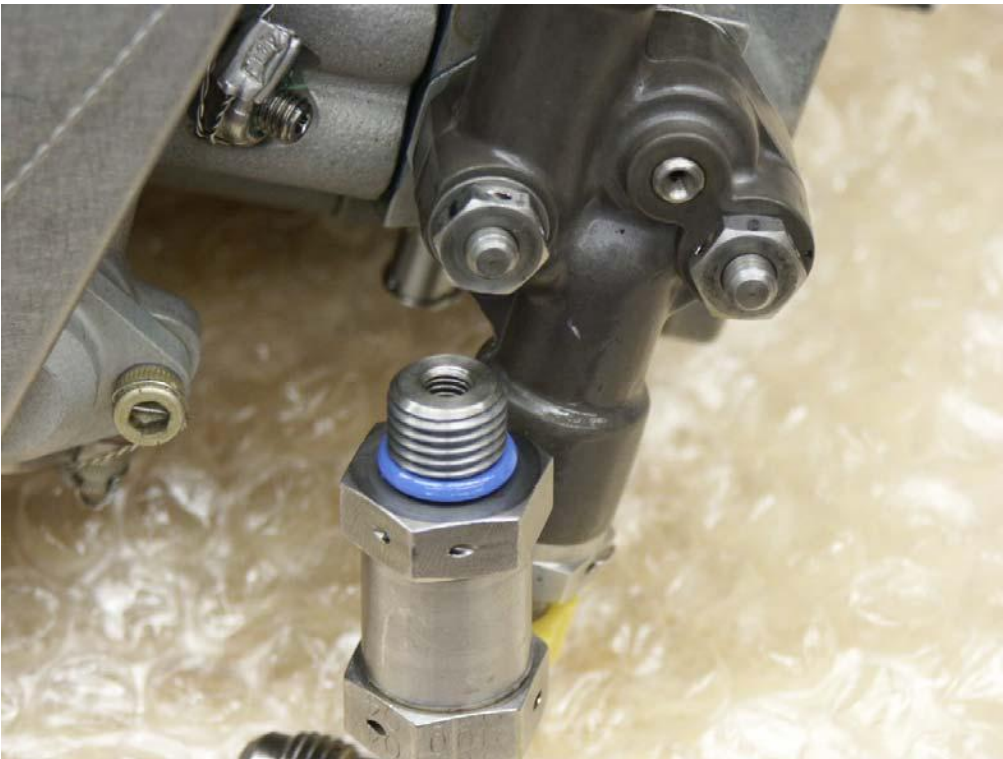
Figure 16 Pc inlet fitting wet with fuel
