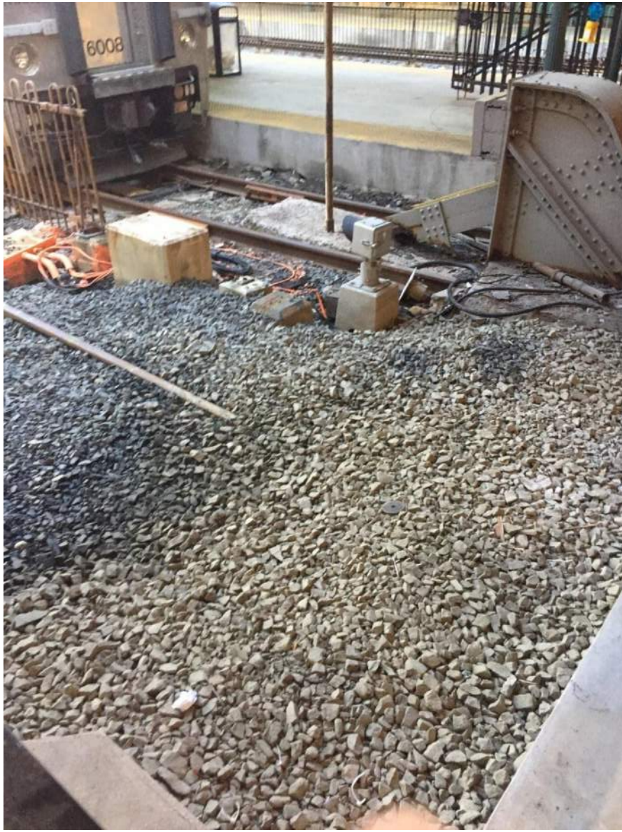
Photo 2 – Track 5 Ballast added, taken May 31, 2017
