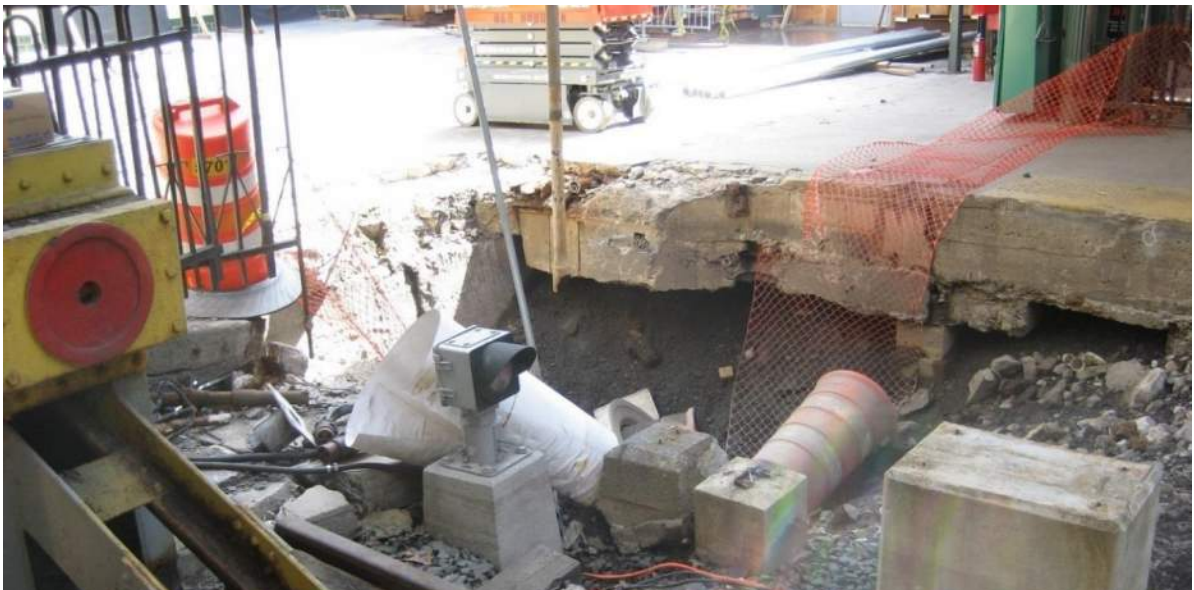
Photo 1 – East End of Track 5, taken March 21, 2017
