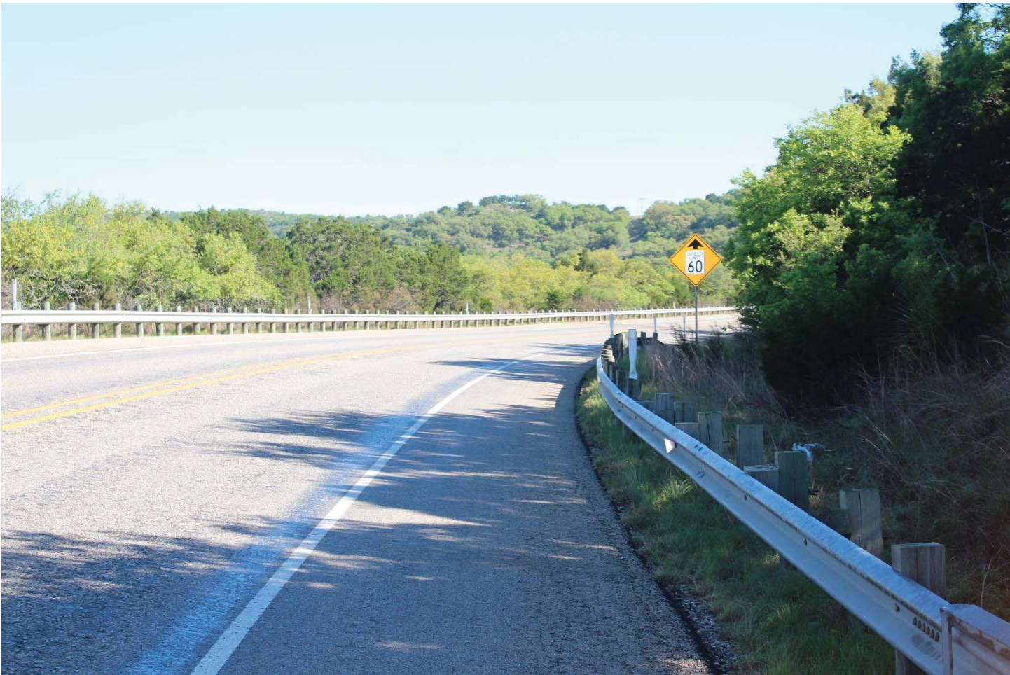
Highway Photo 25 – View of advance warning sign for speed limit change ahead on US 83 from 70 mph to 60 mph.
