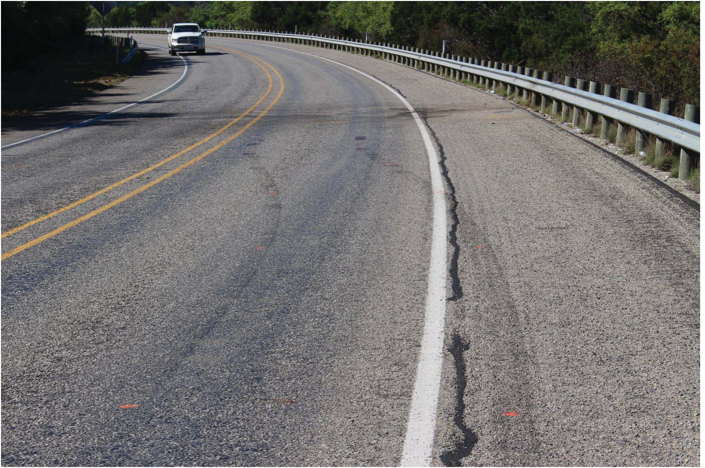
Highway Photo 36 – View of witness vehicle tire friction marks in the southbound lane that skidded to a stop behind the accident bus. Flid stains marking the impact area are just ahead of the tire marks in the photo.
