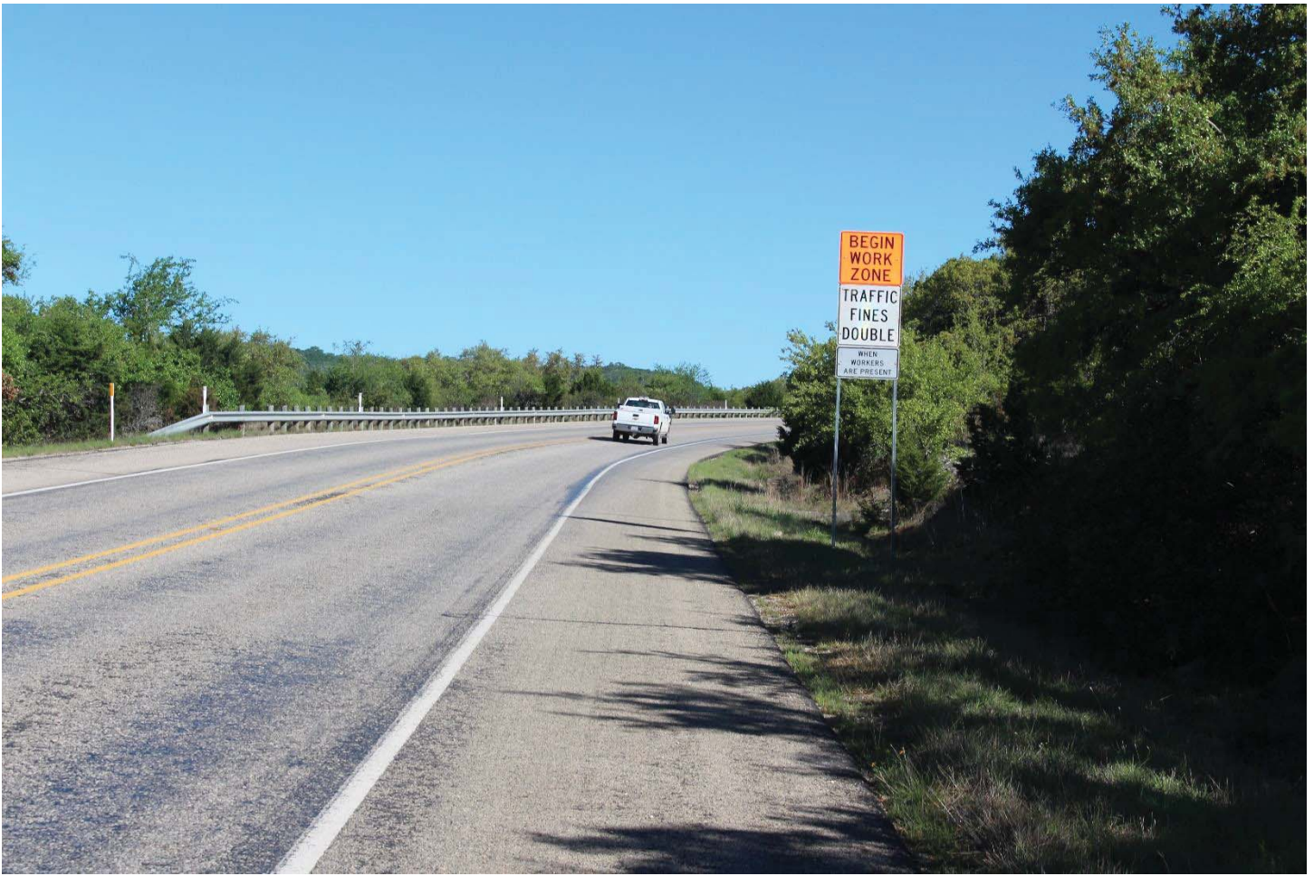
Highway Photo 14 – View of where the work zone began at the beginning of the accident curve
