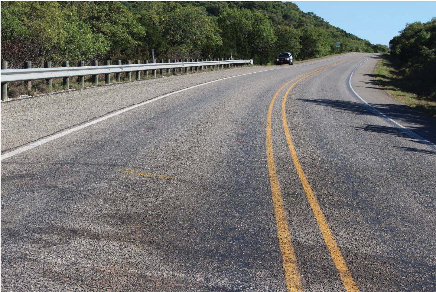
Highway Photo 32 – View of northbound curve ending in the photo background.
