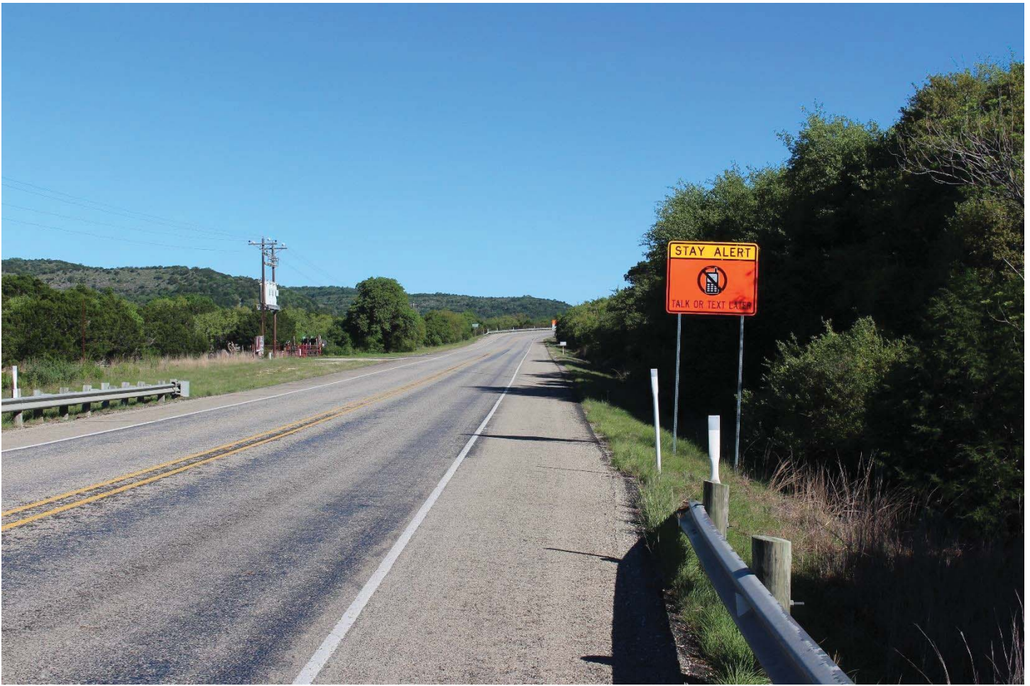
Highway Photo 13 – View of Texas G20.10T sign warning motorist to stay alert and not to text in work zones. The accident curve can be seen beginning approximately 1500 feet away in the photo background.
