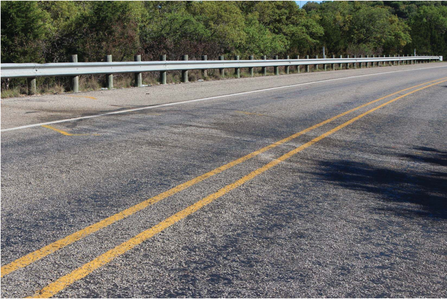
Highway Photo 30 - View of impact area marked by fluid stains and paint markings.
