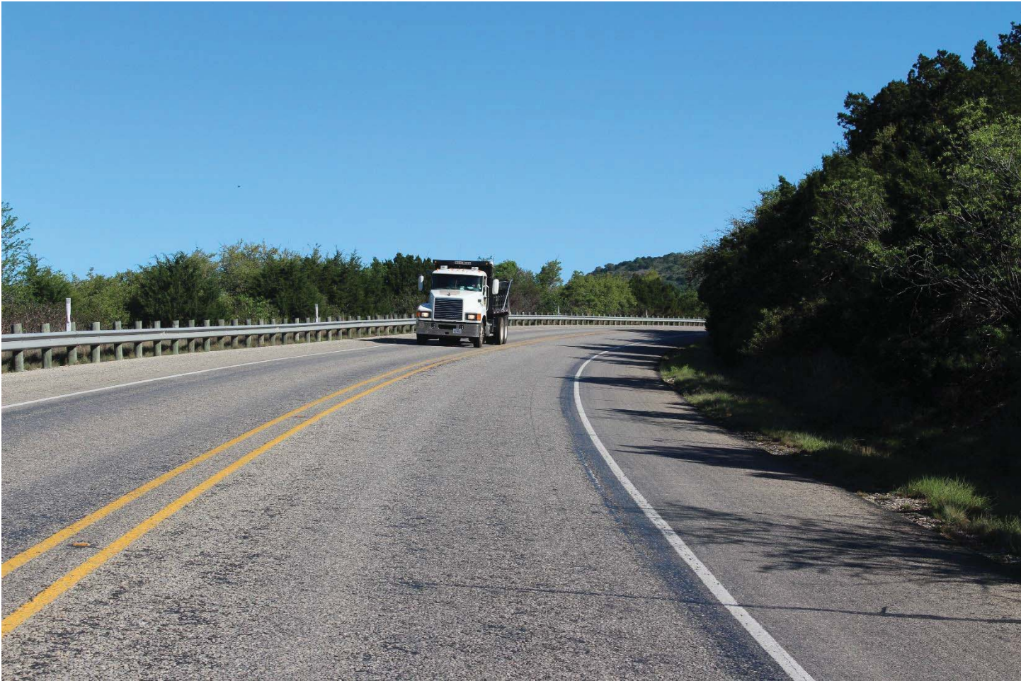
Highway Photo 20 – Northbound view of 4-degree right-hand curve on the uphill grade.
