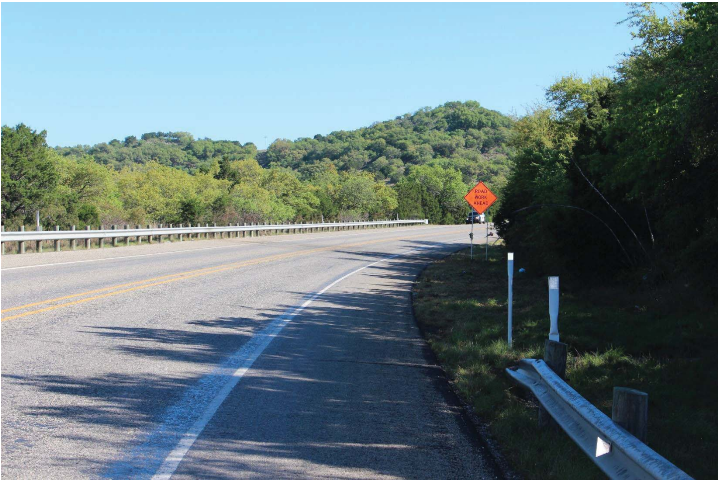
Highway Photo 27 – View of work zone warning sign. Note the impact area can be seen by the pavement discolored by fluid debris on the opposite side of the road across from the sign.
