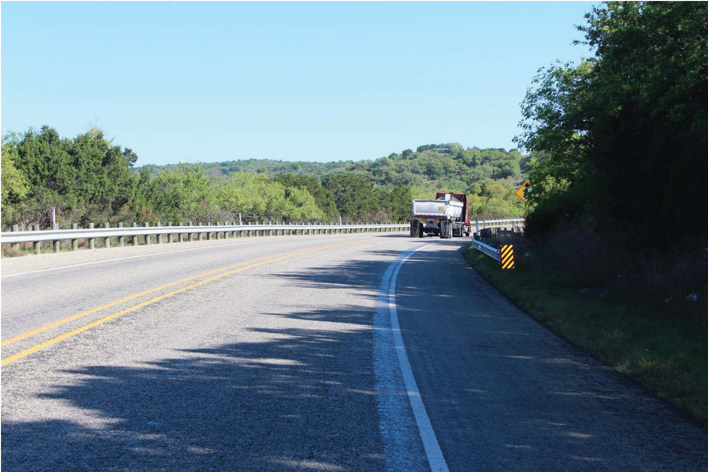
Highway Photo 24 – Continued view of accident curve.
