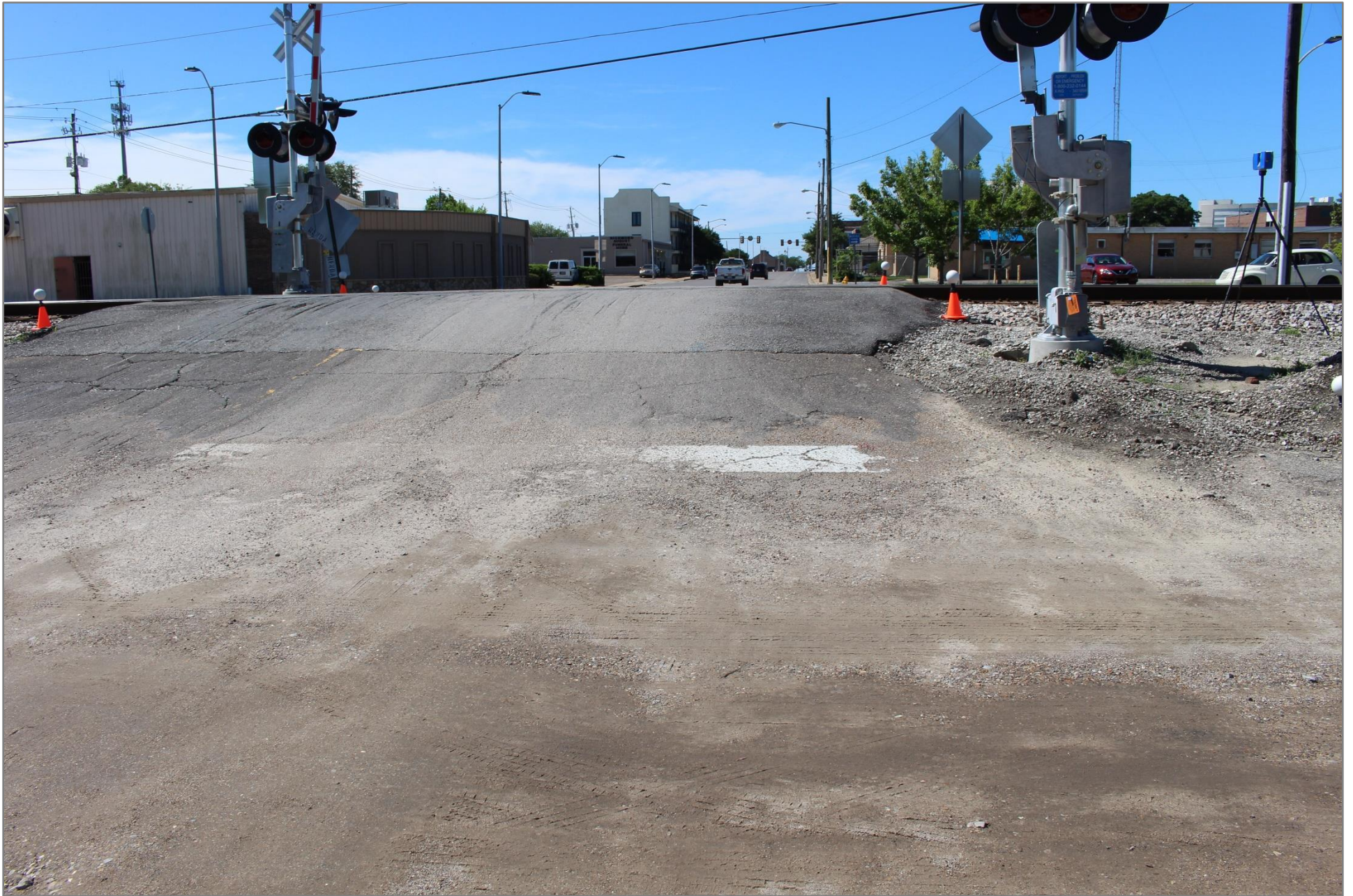
Highway Photograph 9 – Southbound Stop Bar at Grade Crossing – Facing South
