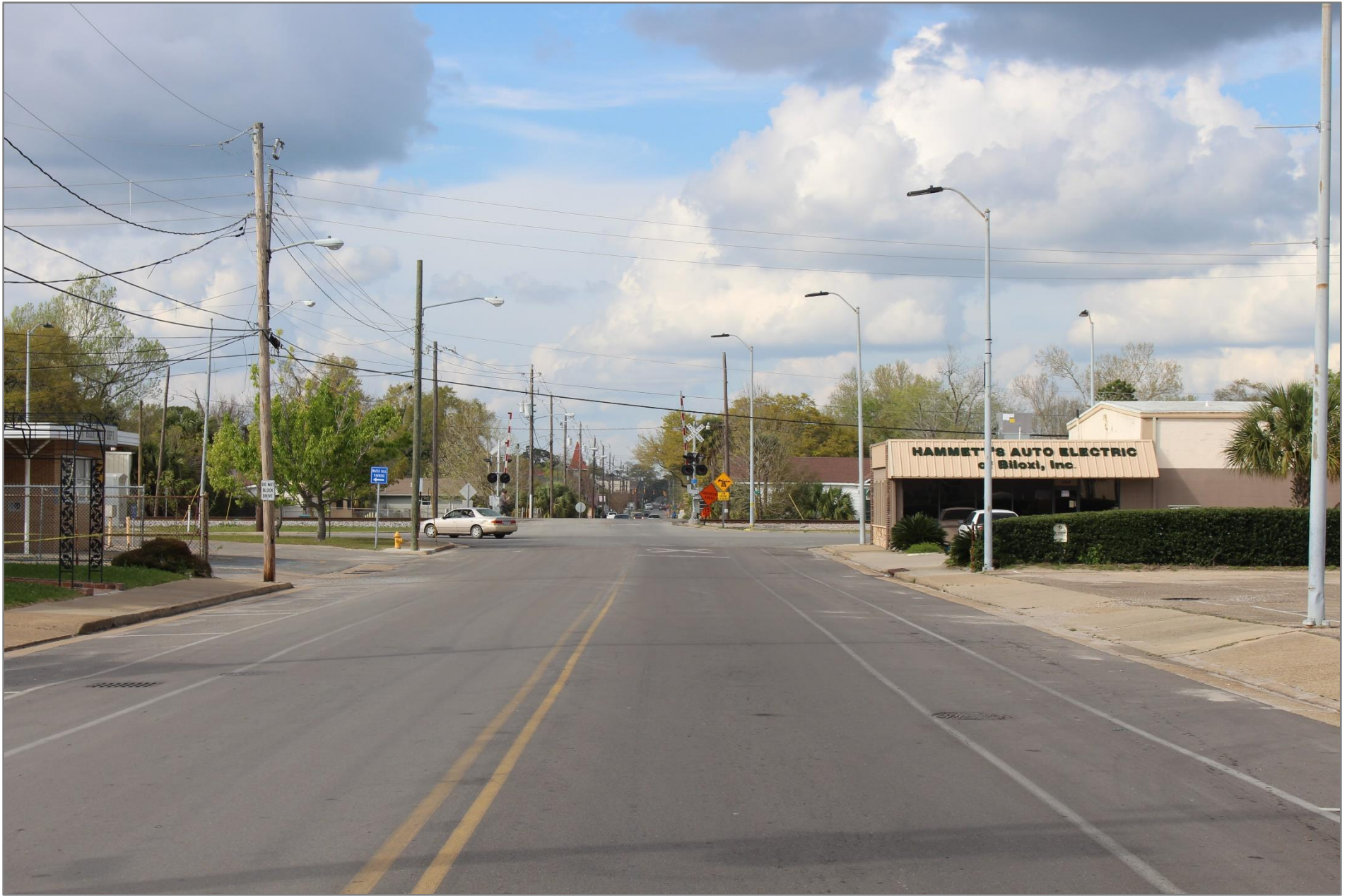
Highway Photograph 1 – Main Street, South of Grade Crossing – Facing North
