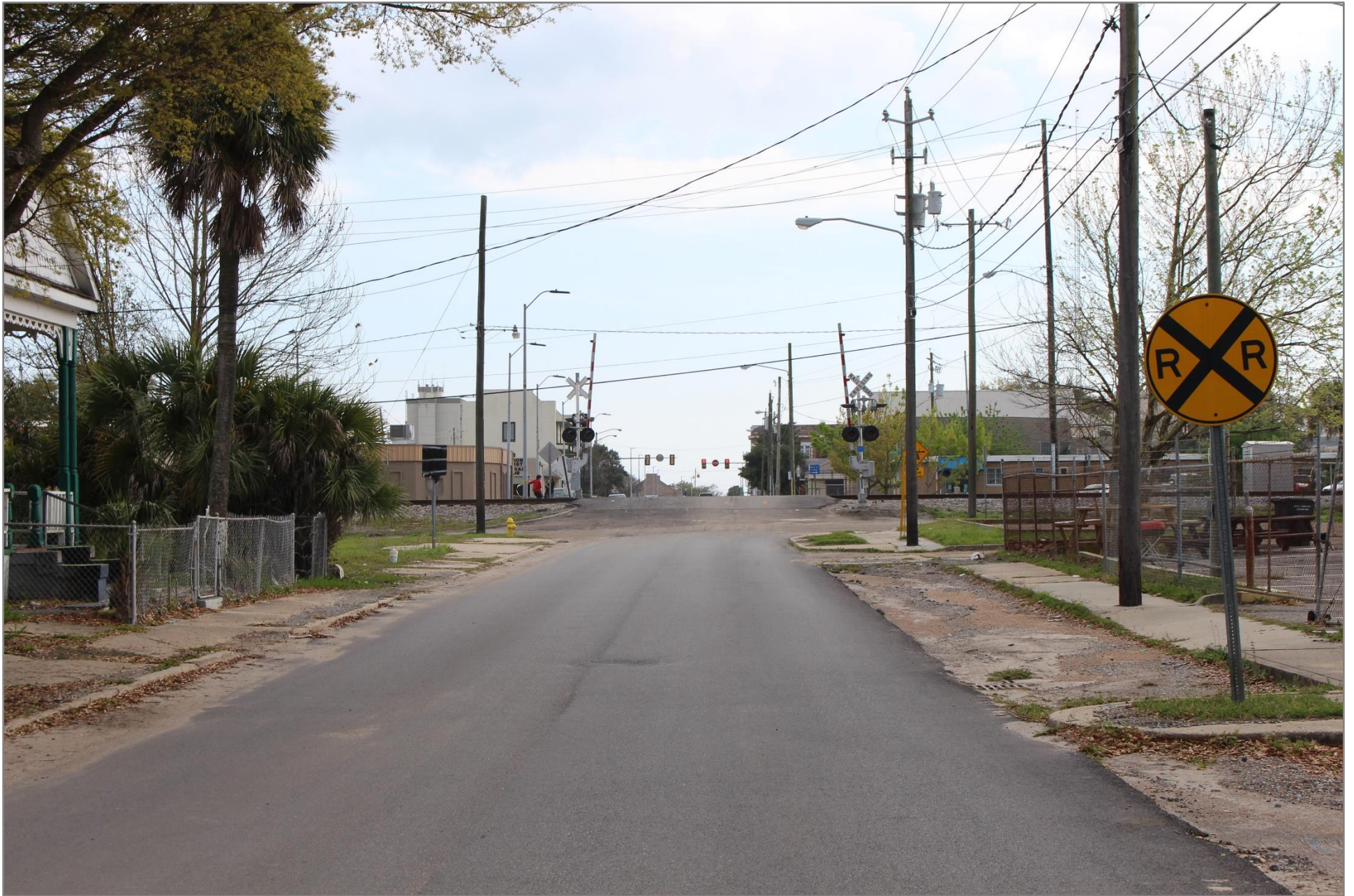
Highway Photograph 6 – Main Street, North of Grade Crossing – Facing South
