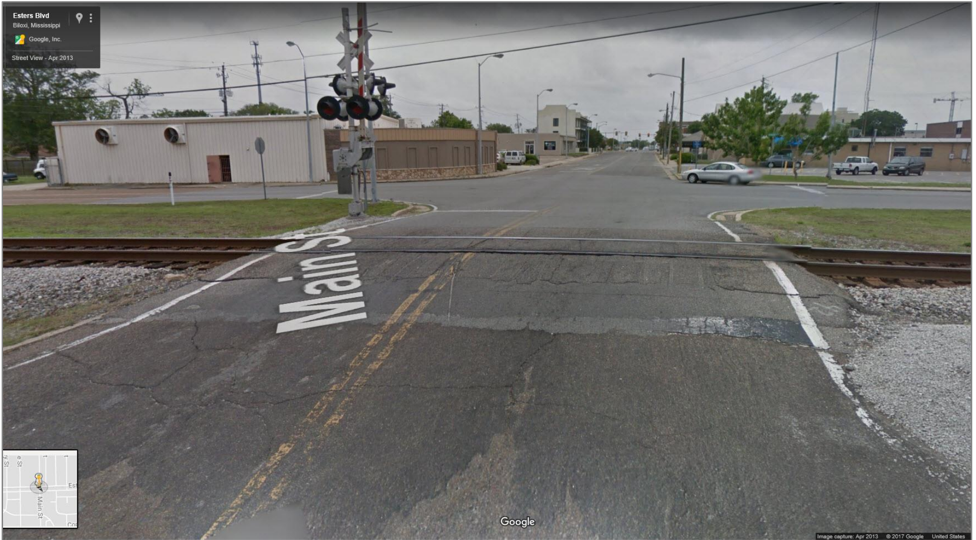
Highway Photograph 15 – Google Maps Street View Image of Main Street Railroad-Highway Grade Crossing dated April 2013 (Source: Google Maps)
