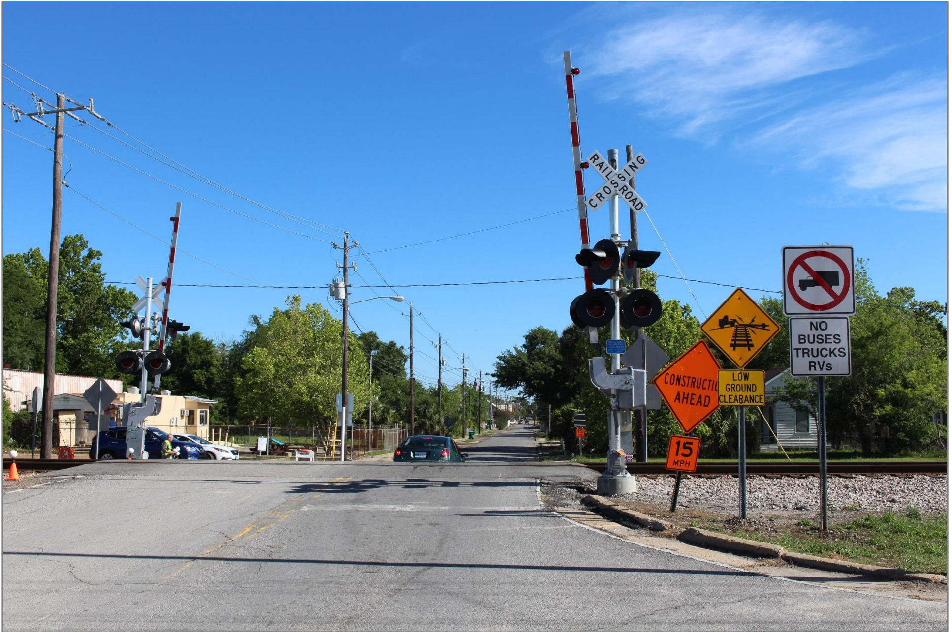
Highway Photograph 10 – Post Mounted Flashing Light Signal System with Automatic Gate, Located in Southeast Quadrant of Grade Crossing – Facing North
