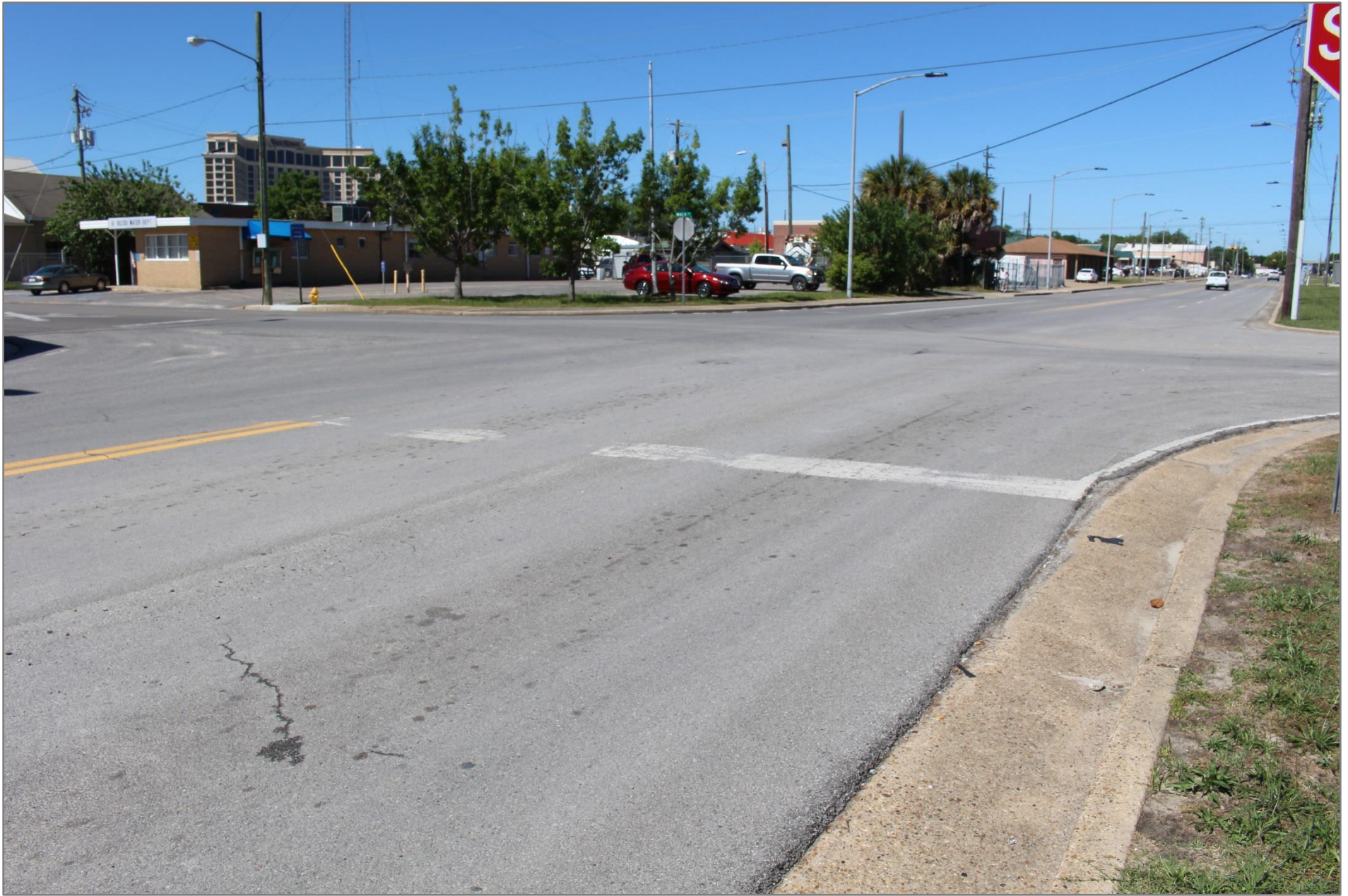
Highway Photograph 2 – Esters Boulevard (South of Tracks) – Facing Southwest
