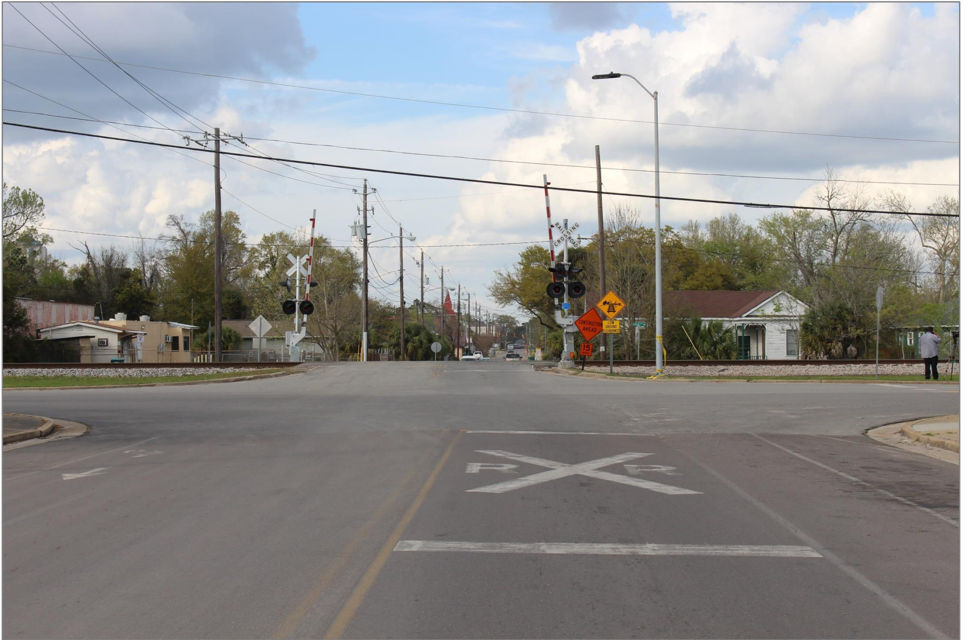
Highway Photograph 7 – Grade Crossing Pavement Marking Symbol on Northbound Main Street, South of Crossing – Facing North
