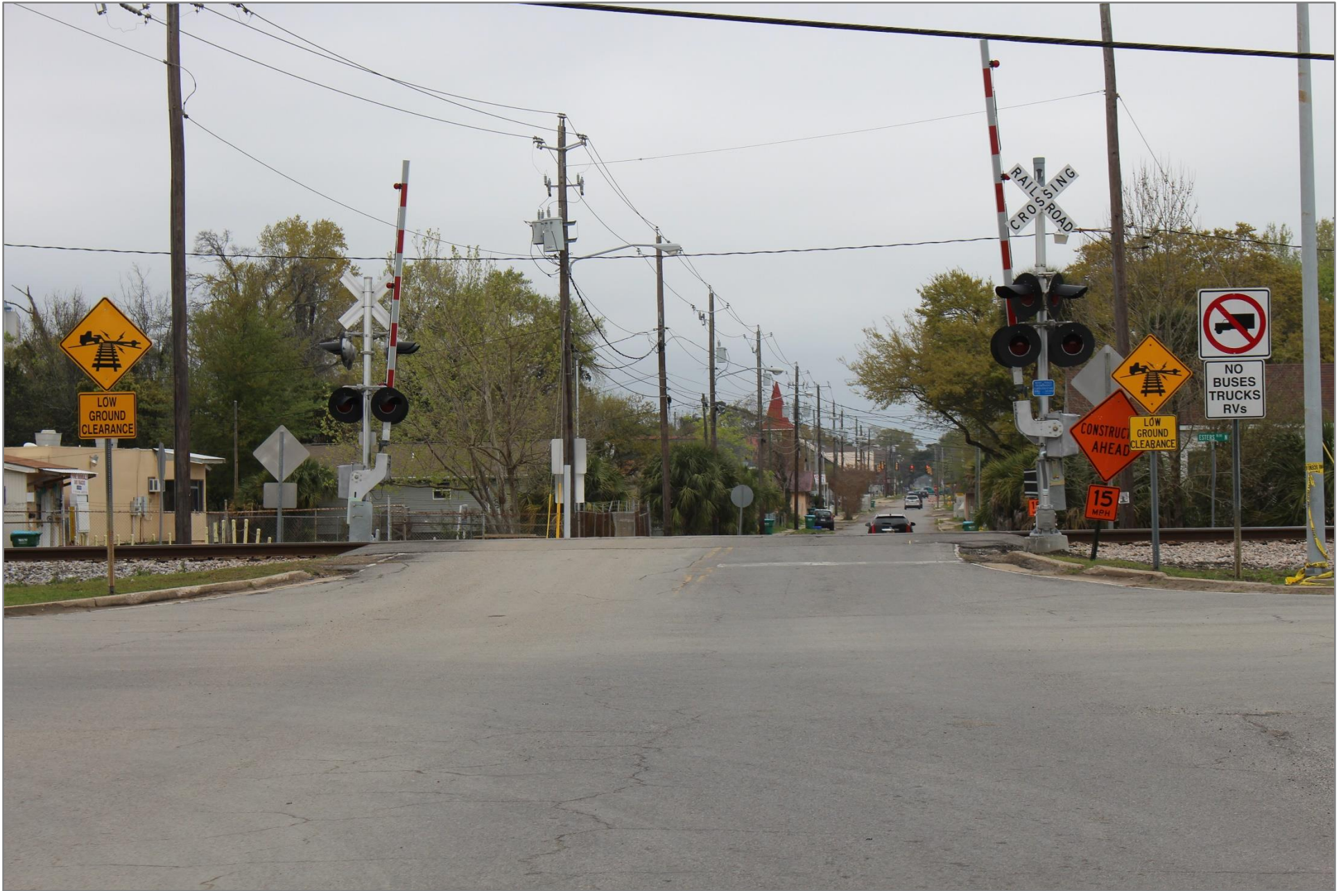
Highway Photograph 19 – Additional Low Ground Clearance Grade Crossing Warning Sign Placed in Southwest Quadrant of Grade Crossing on March 13, 2017
