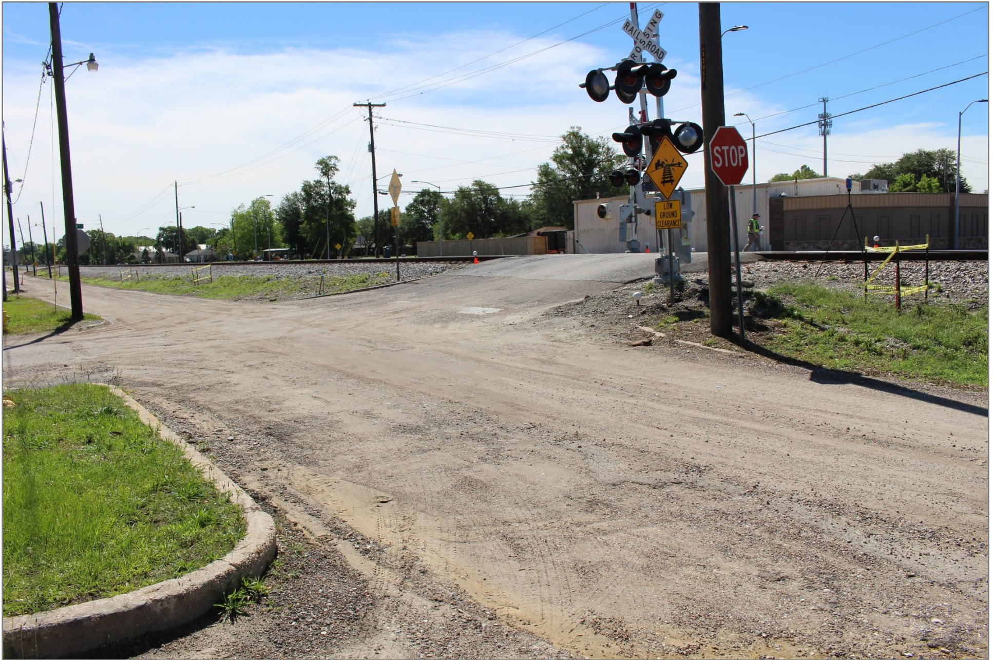
Highway Photograph 5 – Esters Boulevard (North of Tracks) – Facing Southeast
