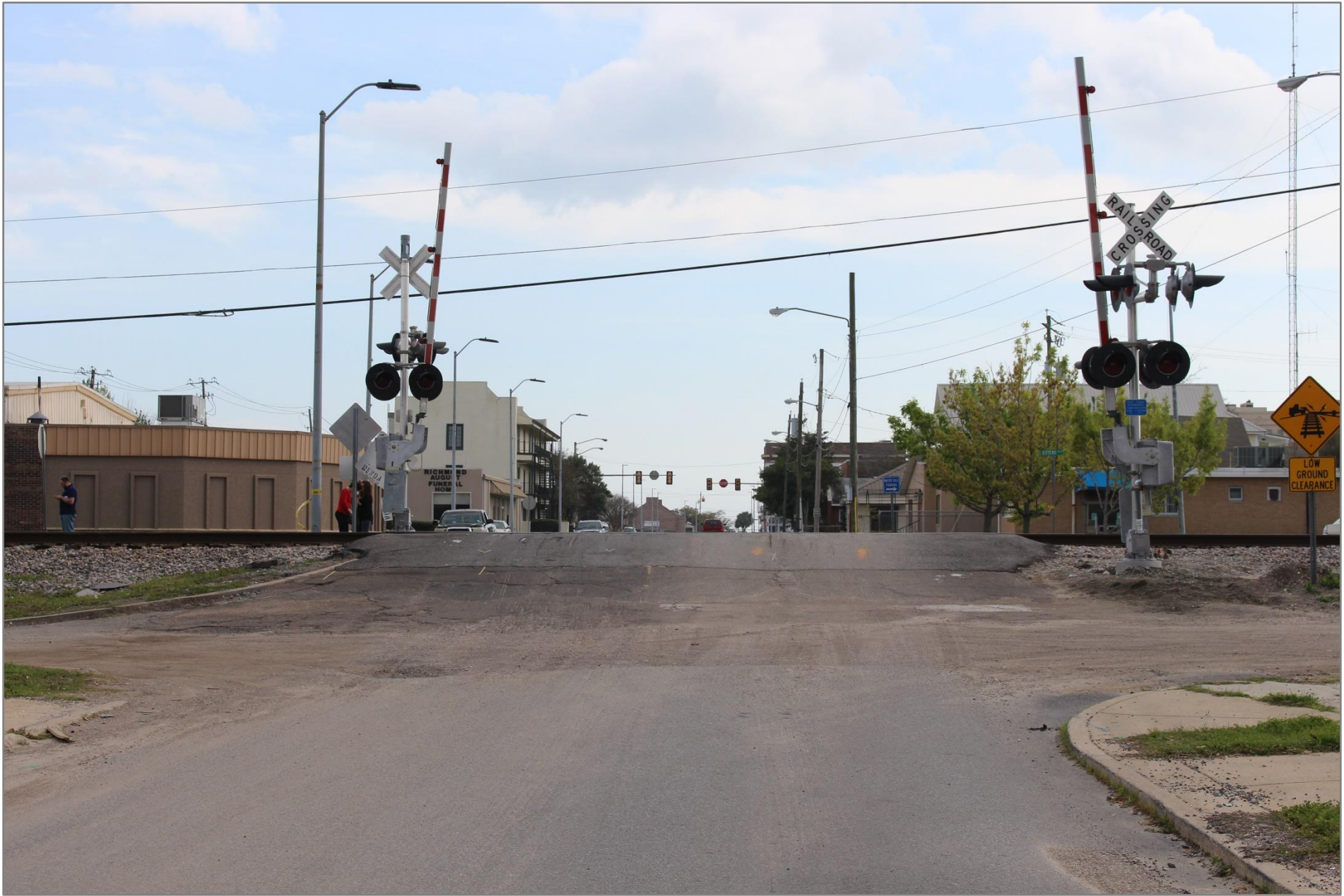
Highway Photograph 4 – Main Street Grade Crossing – Facing South
