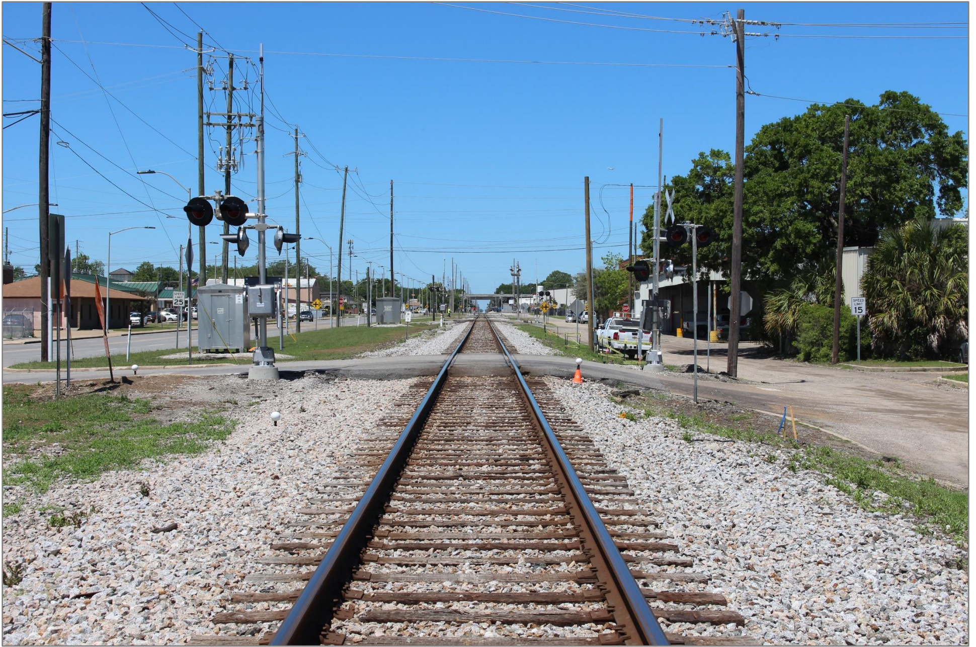
Highway Photograph 11 – Side View of Main Street Crossing – Looking West
