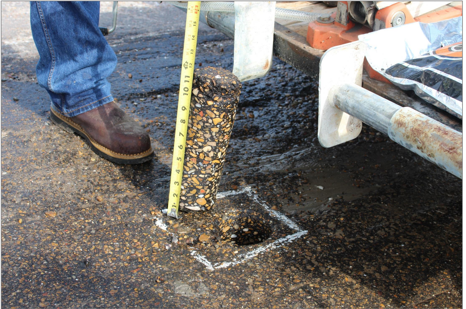
Highway Photograph 16 – Core Sample “C” After Being Removed from Roadway
