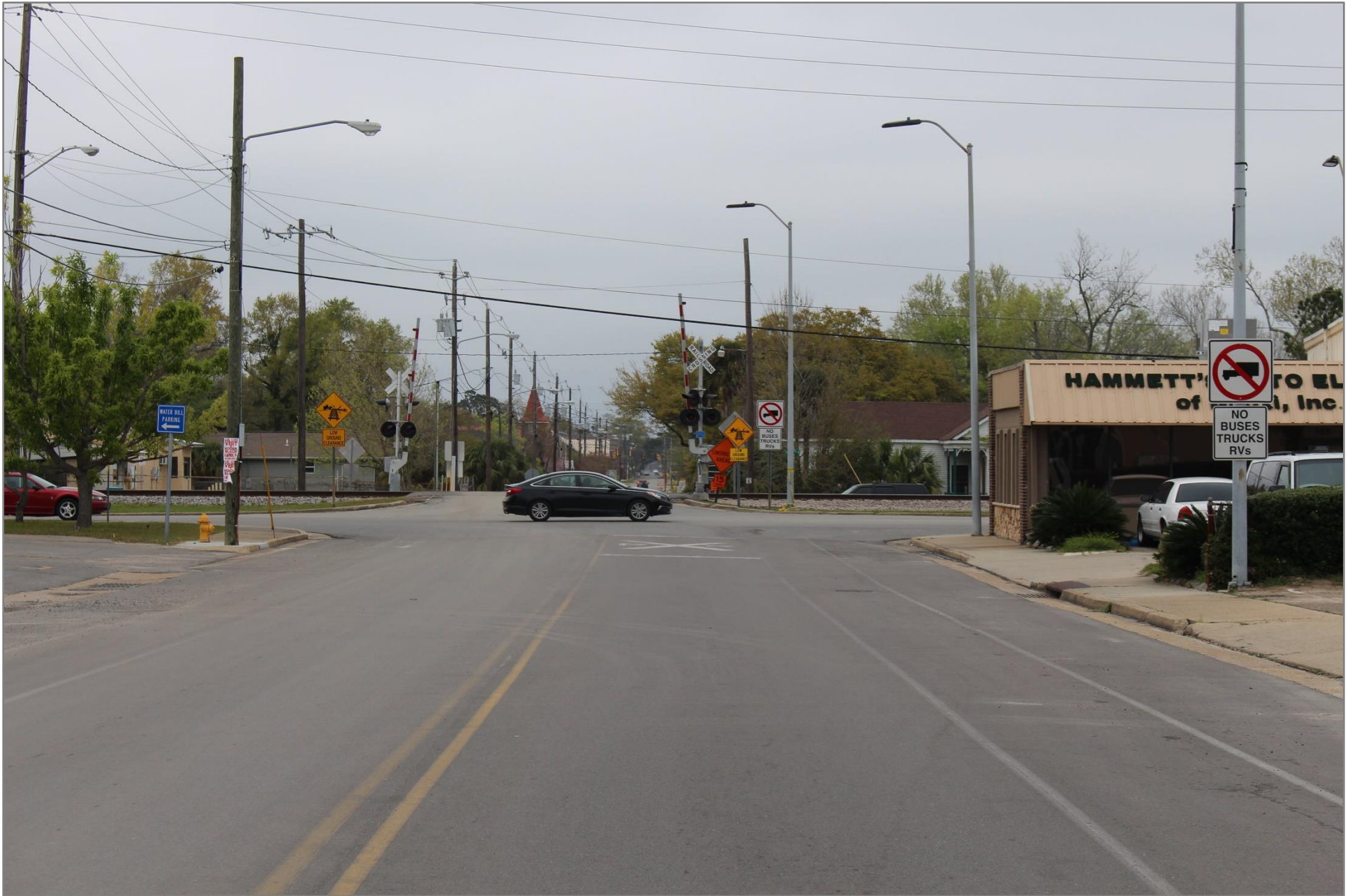
Highway Photograph 18 – No Trucks Selective Exclusion Signs, Placed at Main Street Grade Crossing on March 10, 2017
