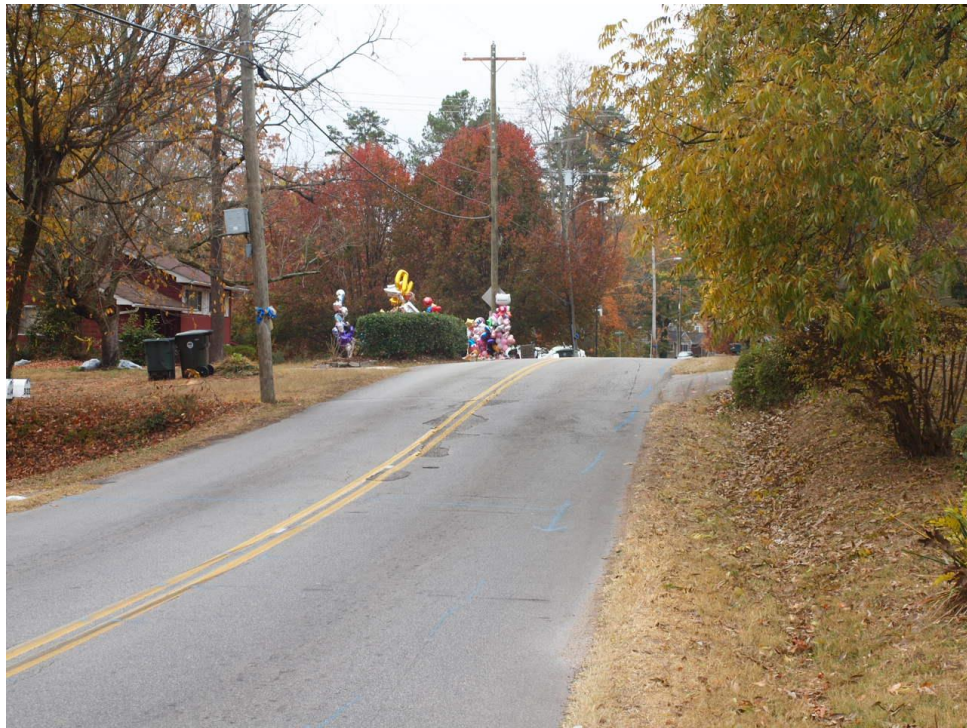
Highway Photograph 9 – View of Talley Road looking in the southbound direction approximately 150 feet prior to the crash location illustrating the upgrade slope of 6.78 percent
