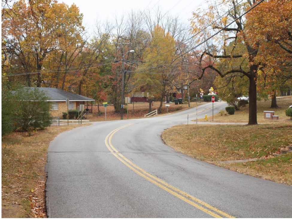
Highway Photograph 8 – View of Talley Road looking in the southbound direction approximately 500 feet prior to the crash location illustrating the horizontal curve to the right
