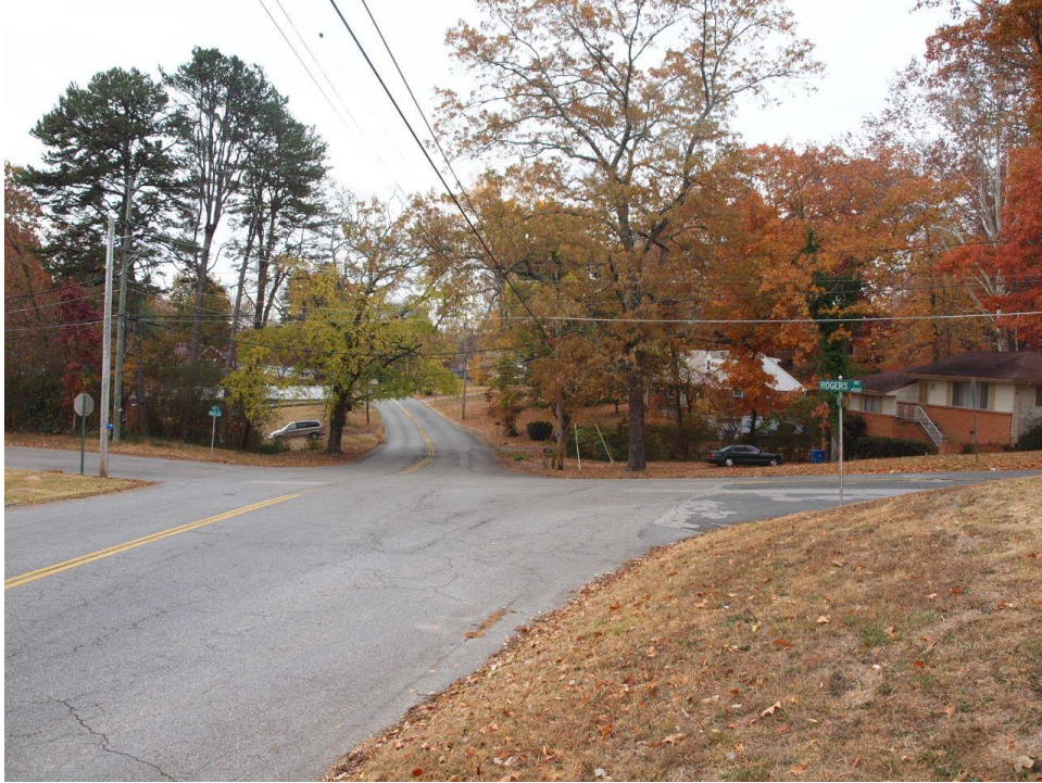
Highway Photograph 6 – View of Talley Road looking in the southbound direction approximately 1,300 feet prior to the crash location illustrating the downgrade slope of 8.17 percent
