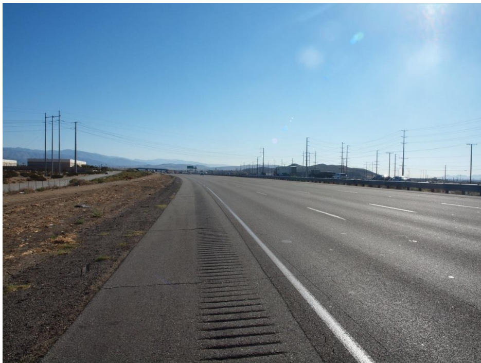
Highway Photograph 2 – View of the westbound travel lanes of I-10 looking to the east from the area of the crash illustrating no obstructions (i.e. shrubbery or signage) were located close to the shoulder that would have obstructed the view of the motorcoach driver as he traversed the 6,000-foot radius curve to the right in the center right lane
