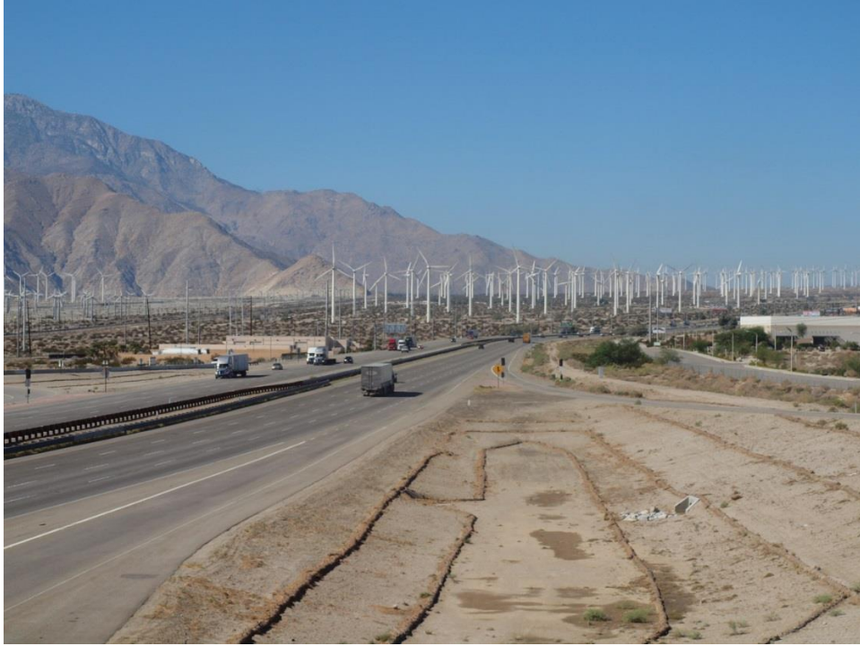
Highway Photograph 11 – View of the westbound lanes of I-10 prior to the crash location standing on the Indian Canyon Drive overpass
