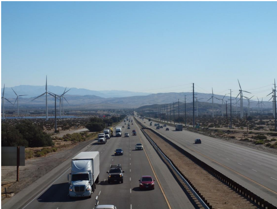
Highway Photograph 12 – View of the westbound lanes of I-10 illustrating the completed utility work in the background standing on the Wall Drive overpass
