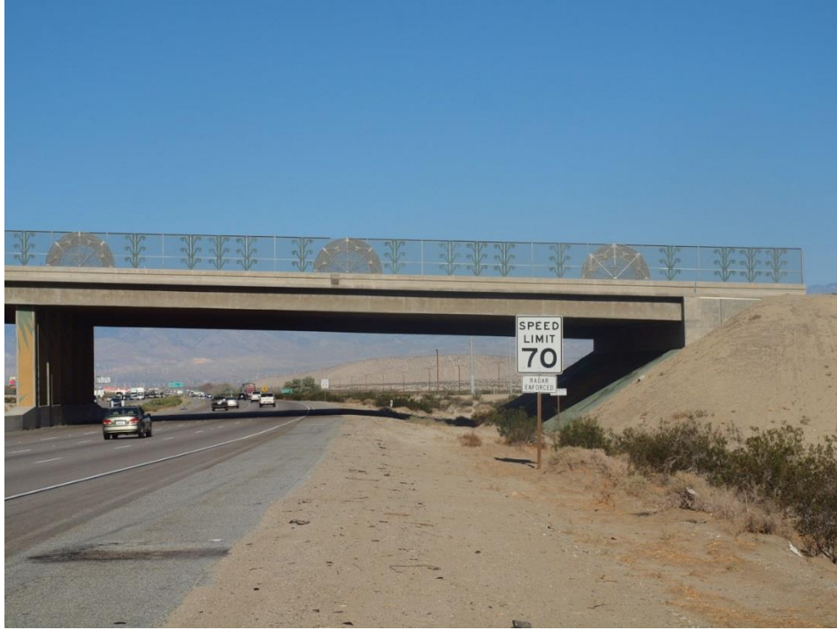
Highway Photograph 13 – View of the posted speed limit sign of 70 miles per hour (mph) in the westbound direction of I-10 prior to the crash location
