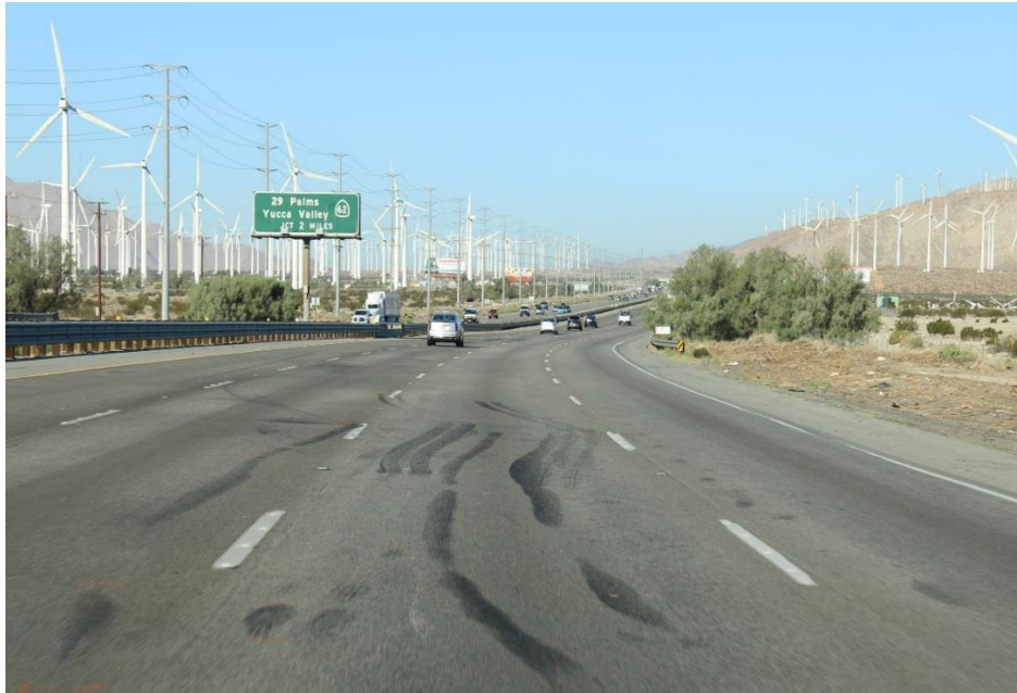
Highway Photograph 1 – View of tire marks and 6,000-foot radius curve to the right in the vicinity of the crash looking in the westbound direction of I-10 in Lane #3
