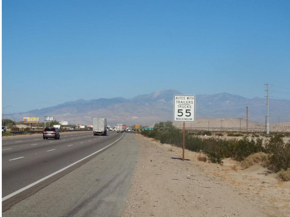
Highway Photograph 14 – View of the maximum speed limit sign for vehicles towing trailers of 55 miles per hour (mph) in the westbound direction of I-10 prior to the crash location
