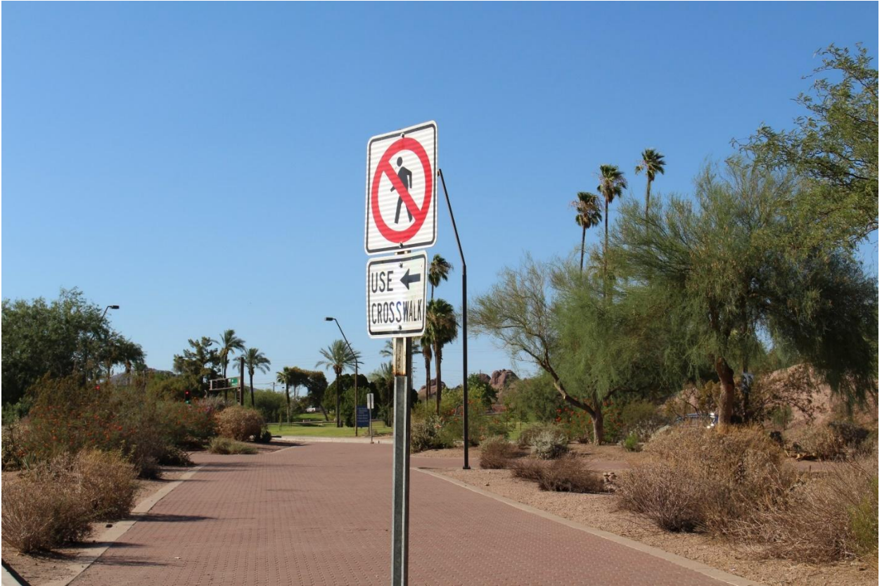
Figure 5 Signs prohibiting pedestrians from crossing South Mill Ave
