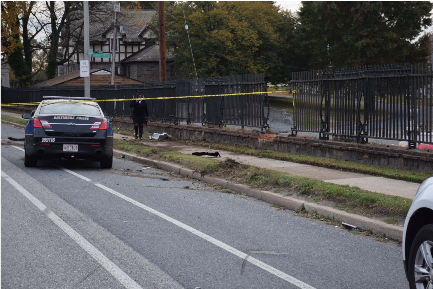
Highway Photo 7 – View of the Mustangs post-crash travel path into the cemetery wall.
