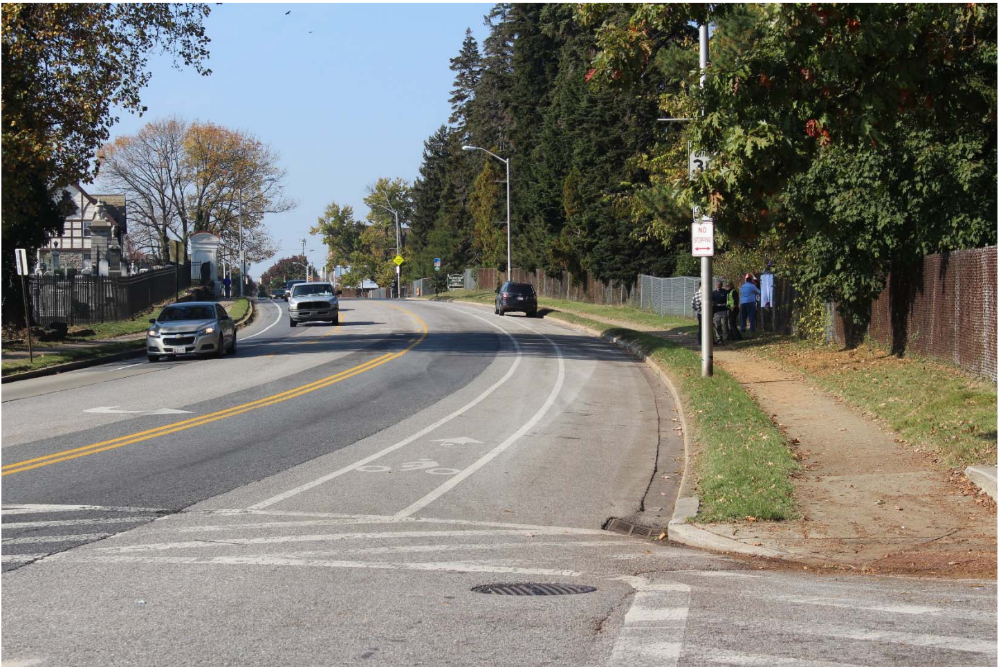
Highway Photo 25 – Westbound view of transit buse’s approach from Morley street. Note the slope and curvature of the roadway. The impact area is near where the curve begins in the area covered by the shade of the trees.
