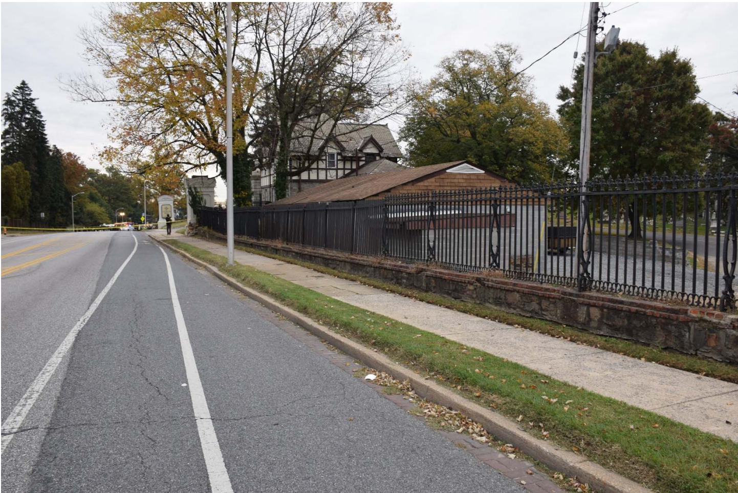
Highway Photo 19 – Continued view looking east on Frederick Avenue showing the buses on the other side of a slight hill crest past the entrance to the cemetery.
