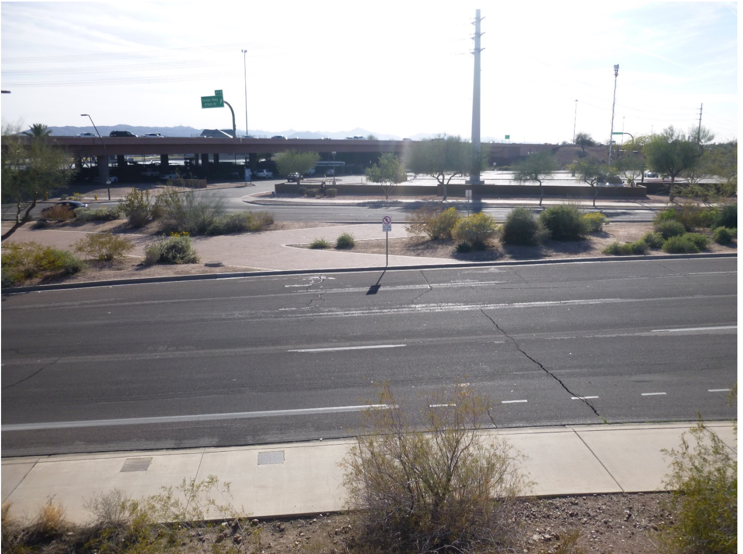
Highway Photo 9 – Additional view of North Mill Avenue looking where the impact occurred in the right-hand lane perpendicular to the drainage inlet on the left in the photo.
