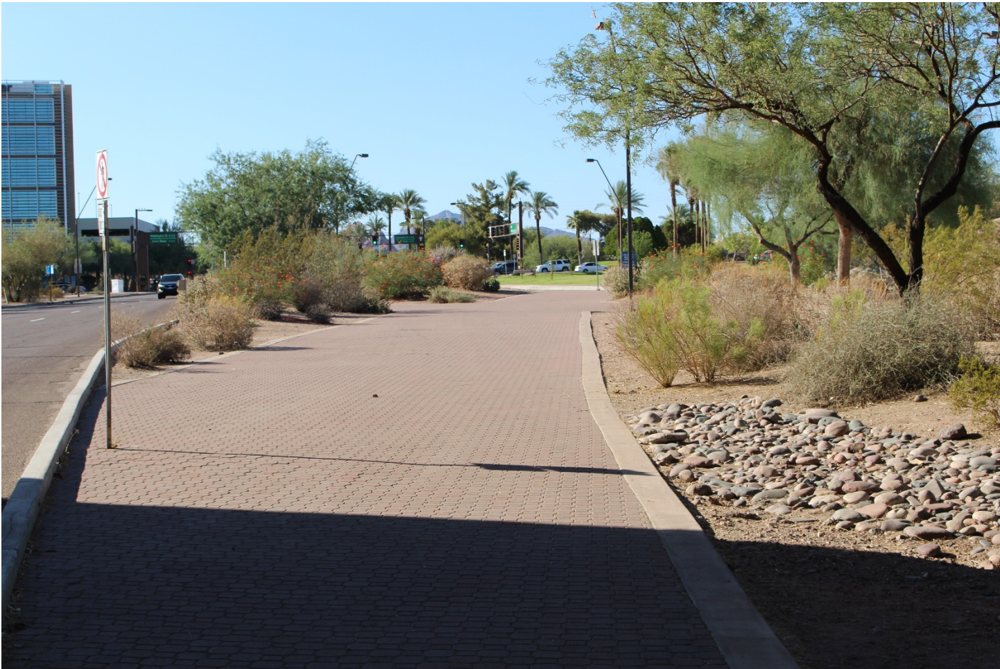
Highway Photo 2 – Continued view of pedestrian’s path in the median toward N. Mill Avenue. Note the sign facing outward in the left side of the photo that prohibits pedestrians from crossing S. Mill Avenue into the median area.
