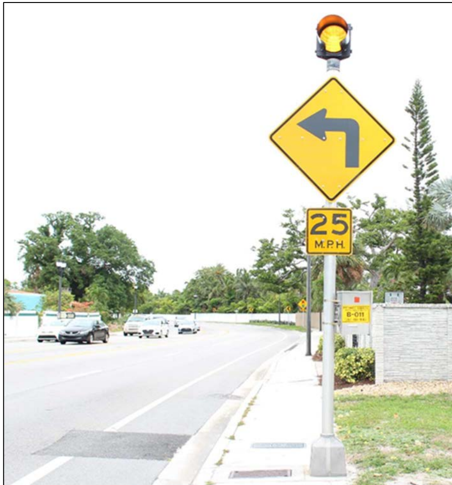
Figure 5: Photograph depicting arrangement of southbound warning signs preceding the curve on which the collision occurred. Image has been cropped.
