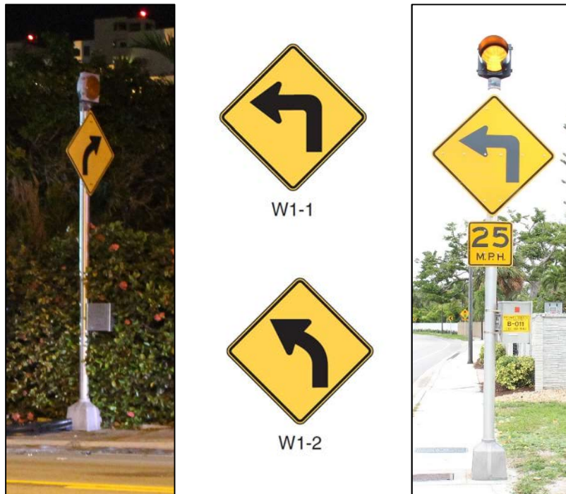
Figure 2: Depicted above are photographs and illustrations of the horizontal alignment warning provided in advance of the curve. The left image (provided by FLPD investigators) faces northbound traffic, while the right image (provided by NTSB investigators) faces southbound traffic.
