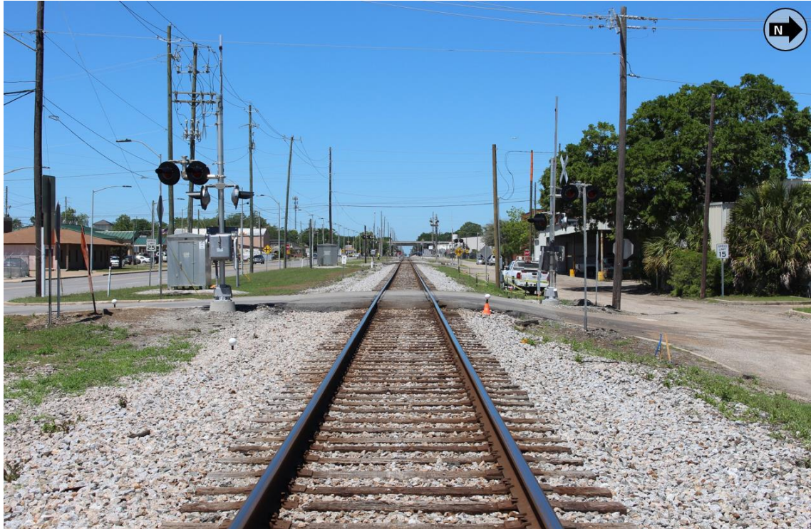
Figure 9: Photograph Showing the Side Profile of the Main Street Grade Crossing – Looking West
