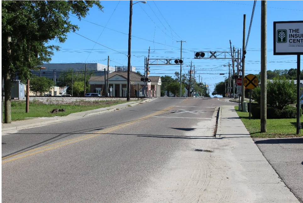
Figure 15: Photo of the Approach Slopes at the Porter Avenue Crossing
