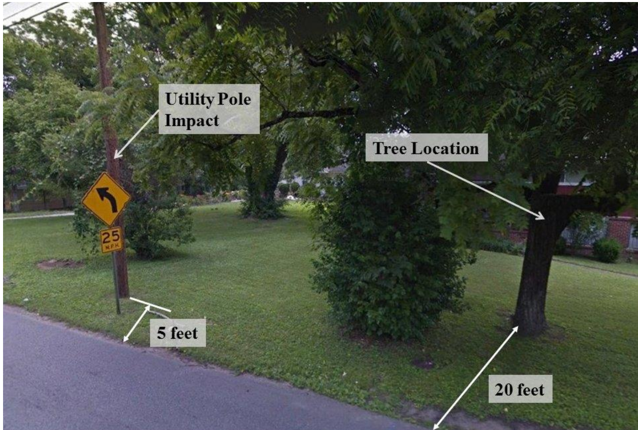
Highway Photograph 5 - Utility pole impact and tree location in relation to the edge of pavement for Talley Road (Source: Google Earth Street View modified)
