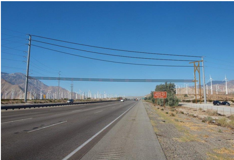
Photograph 3 – Illustration depicting Stage 2 utility work
