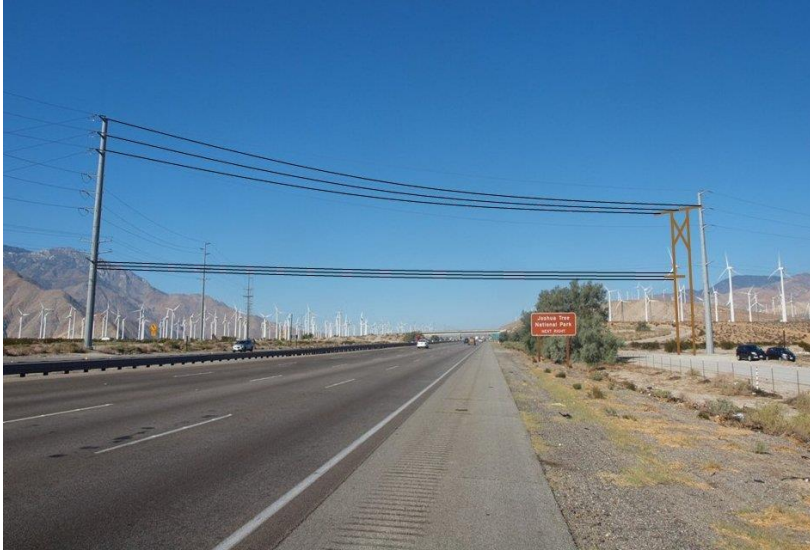
Photograph 2 – Illustration depicting Stage 1 utility work
