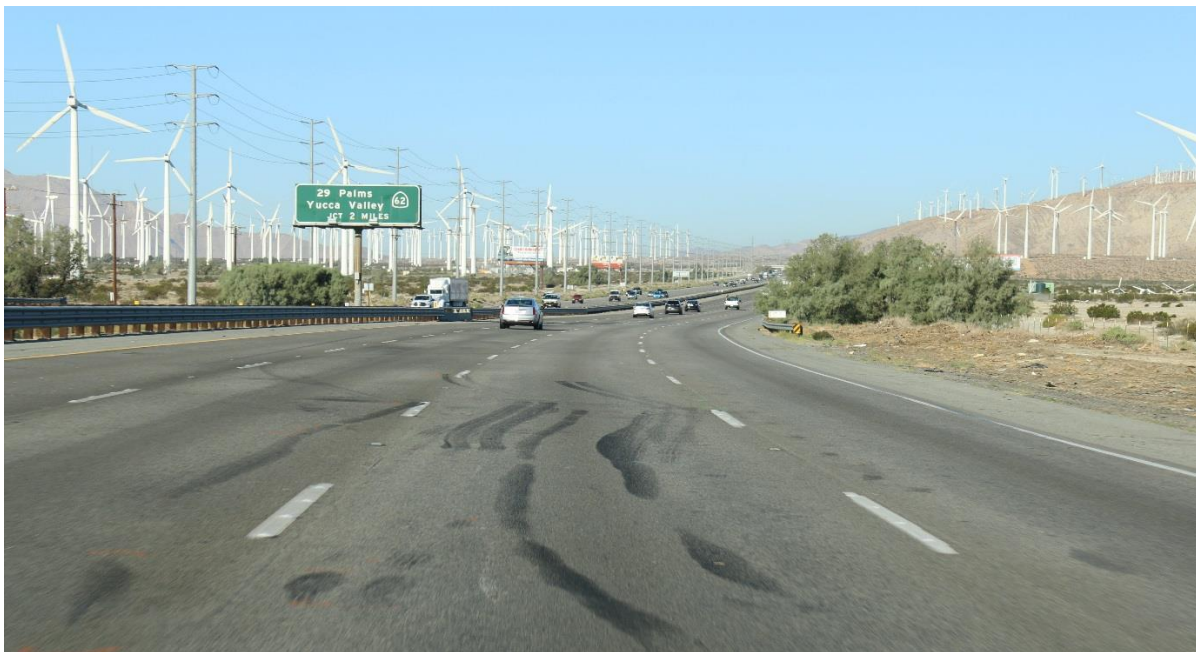
Highway Photograph 1 – View of tire marks and 6,000-foot radius curve to the right in the vicinity of the crash looking in the westbound direction of I-10 in Lane #3
