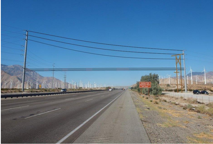
Photograph 4 – Illustration depicting Stage 3 utility work
