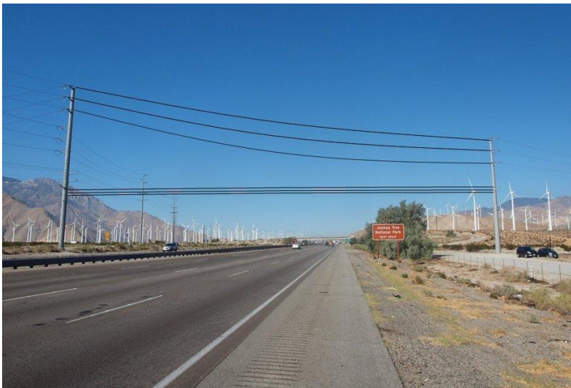
Photograph 5 – Illustration depicting Stage 4 utility work
