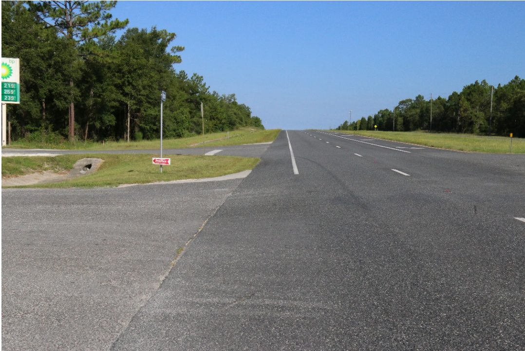
Figure 3. View looking west of the US-27A eastbound travel lane approaching the intersection with NE 140th Court. This is the travel path of the car.
