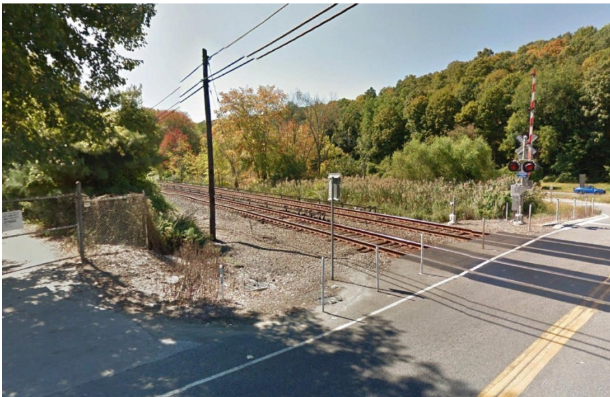
Photograph 2 – Another view of the Green Lane grade crossing looking to the southeast in Mount Kisco, New York in which raised delineator posts have been used to prevent vehicles from inadvertently turning onto the tracks
