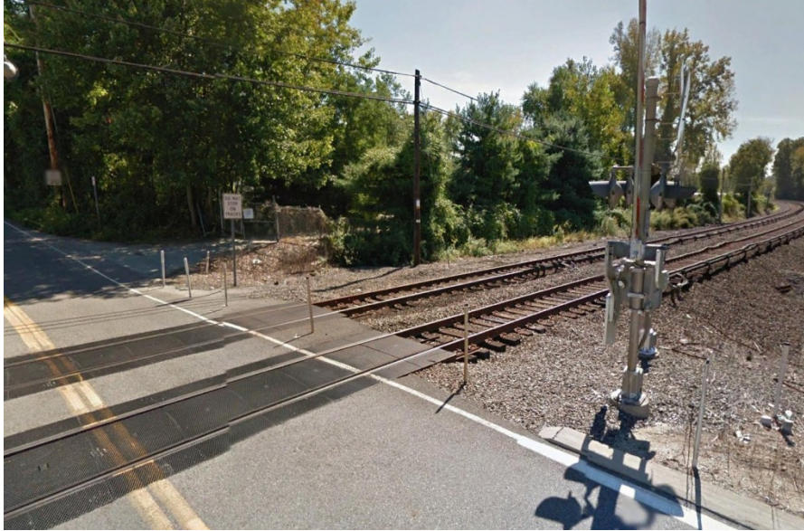
Photograph 1 – View of the Green Lane grade crossing looking to the northwest in Mount Kisco, New York in which raised delineator posts have been used to prevent vehicles from inadvertently turning onto the tracks
